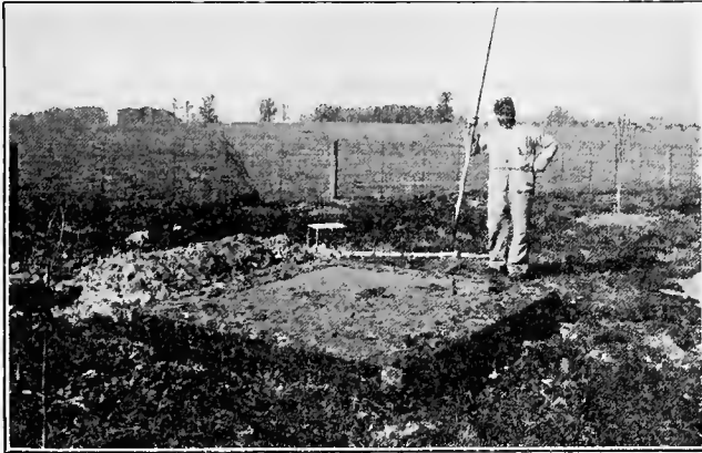
SCREEN PIT OVERFLOWING THROUGH OMISSION OF CLEANING.
