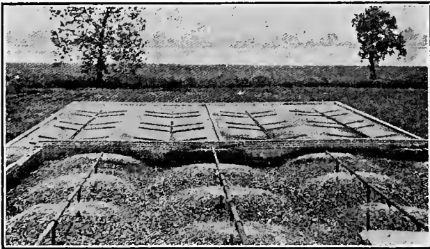
SPRINKLING FILTER WITH INVERTED NOZZLES.
