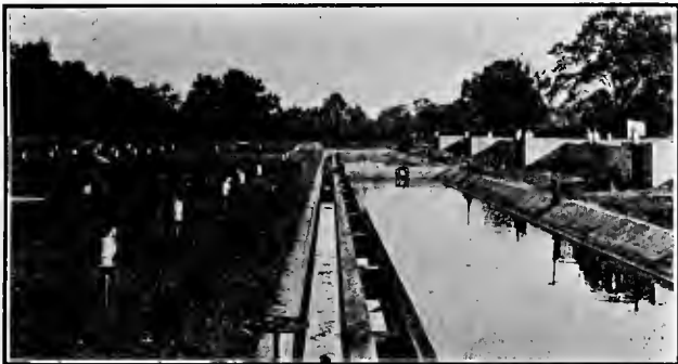
SETTLING BASINS FOR CONTACT EFFLUENT.
