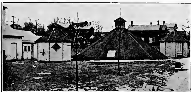
SEWAGE TREATMENT PLANT AT RED BANK.
