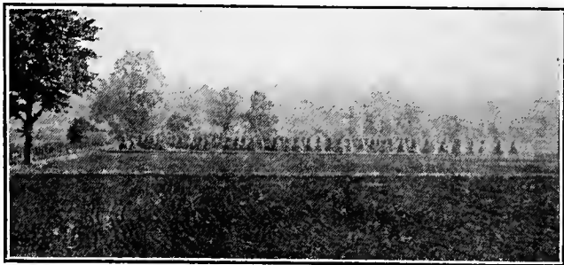
LAND FILTRATION AREA, RECEIVING RAW SEWAGE. Kept plowed and free from vegetation—corn is sometimes raised on the idle beds.
