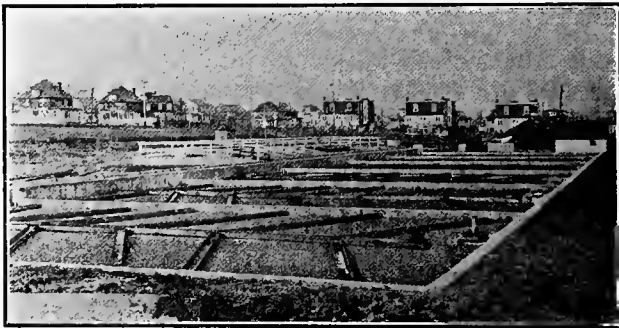
CONTACT BEDS WITH WOODEN TROUGH DISTRIBUTION.
