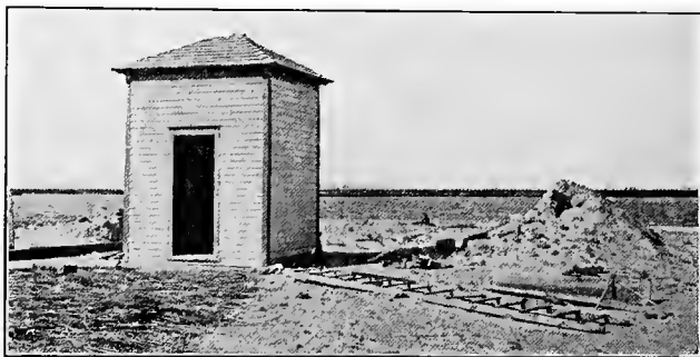
FIRST CHLORIDE OF LIME SEWAGE DISINFECTION PLANT IN NEW JERSEY, BUILT IN 1909.
