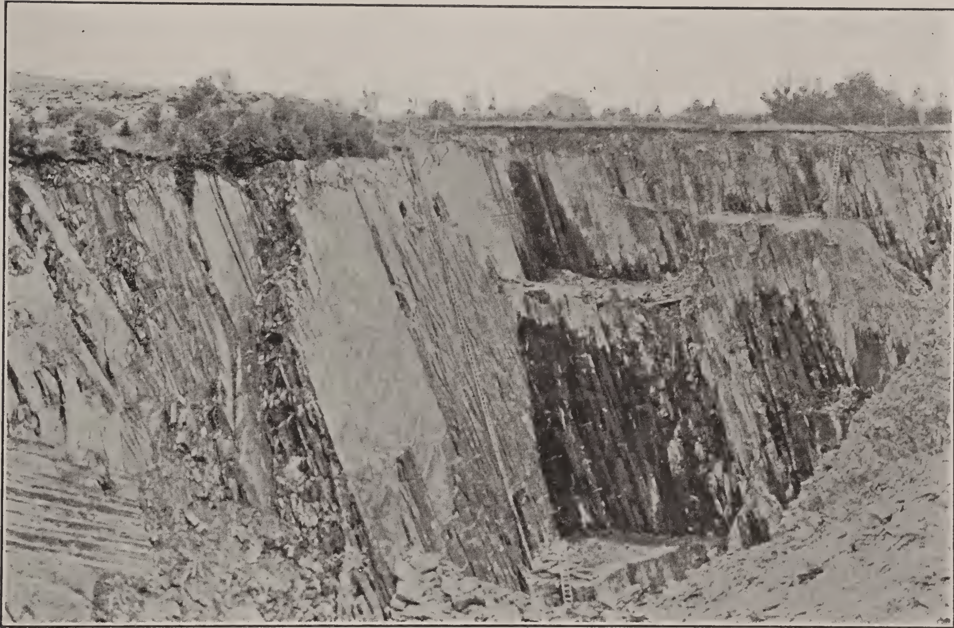
Difficulties that must be overcome in an important slate quarry at Brownville, Me. The photograph shows the pit in which are forty-two beds of slate alternating with an equal number of fissile sandstone known as quartzite. The wall to the left is almost a solid bed of this peculiar sandstone held together by the natural mineral cement of quartz.
