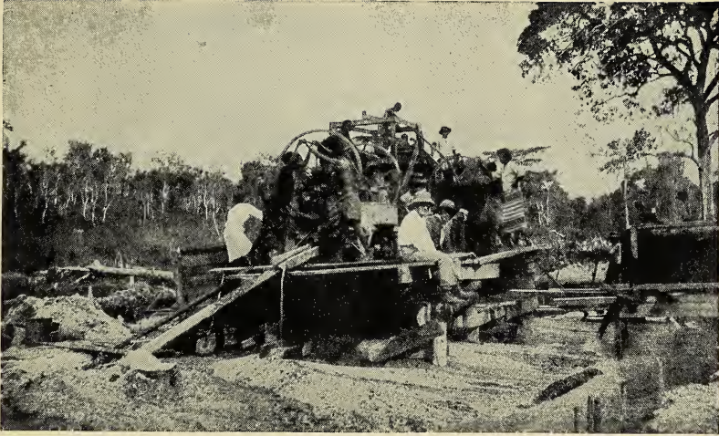
WASHING OUT GRAVEL
