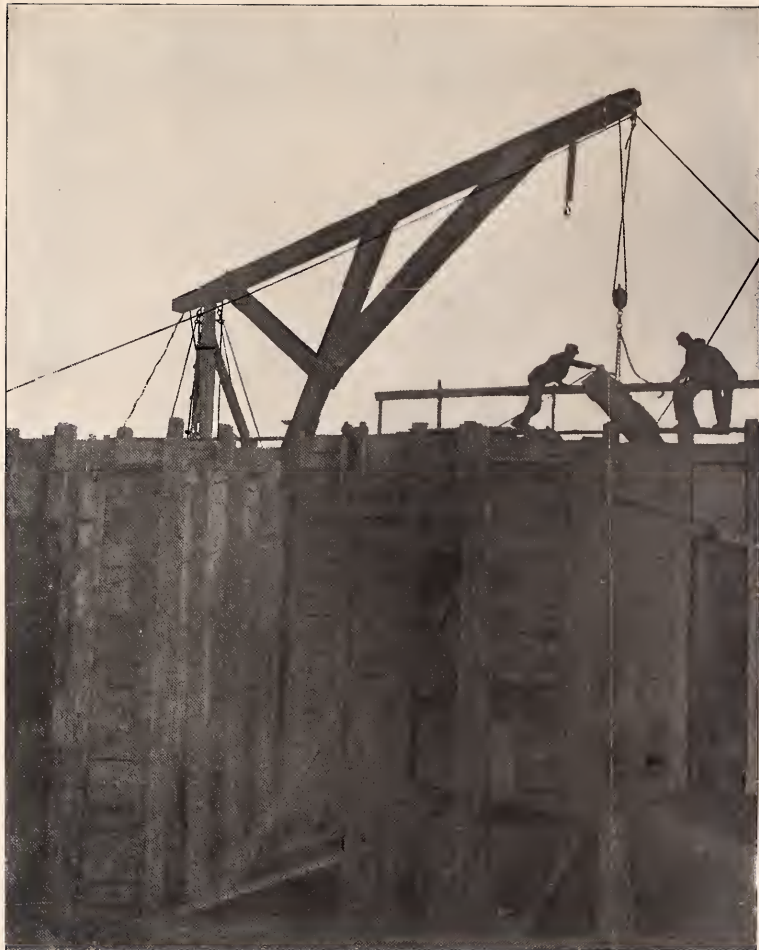
FIG. 4. SHOWING MANNER OF FILLING MOLDS
