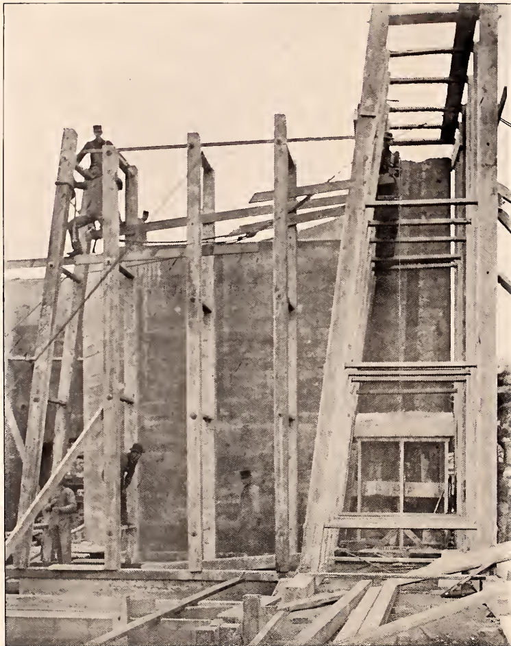
FIG. 2 SHOWING CONSTRUCTION OF MOLDS.
