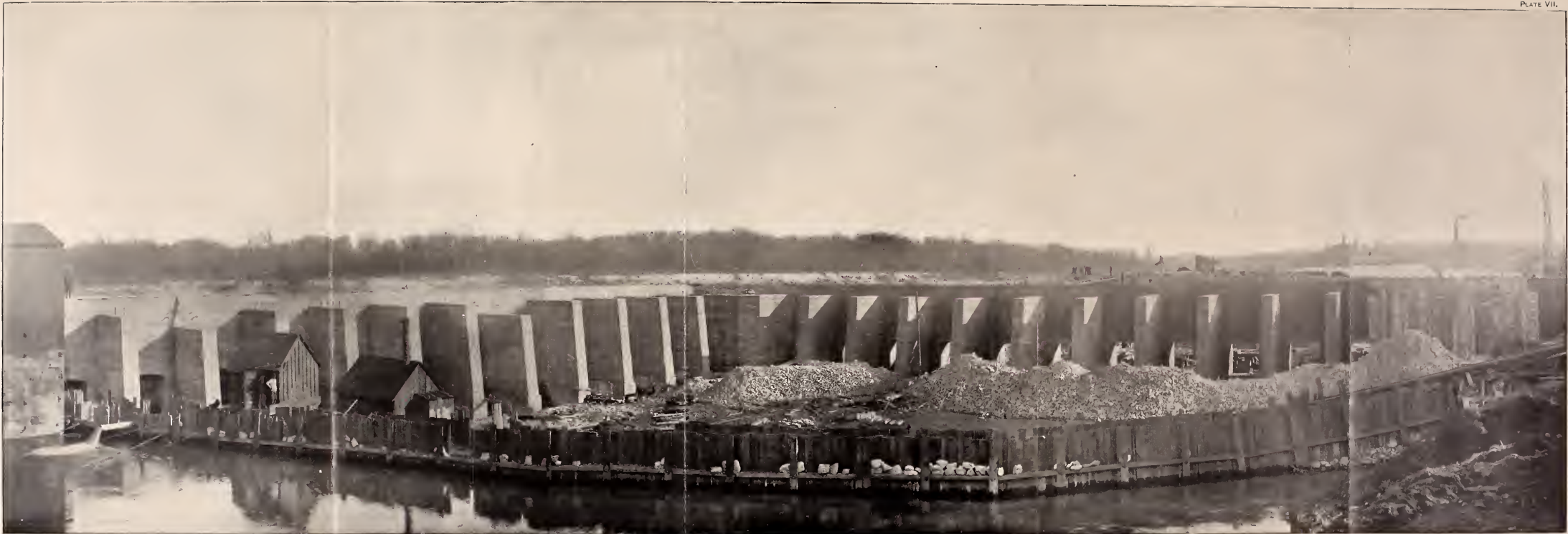
REAR VIEW OF COMPLETED WALL. PART OF MOLDS STILL IN PLACE.
