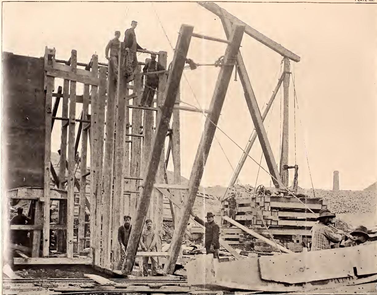
FIG. 1. SHOWING CONSTRUCTION OF MOLDS.
