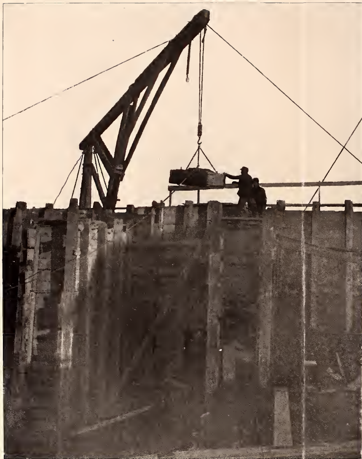
FIG. 3. SHOWING MANNER OF FILLING MOLDS.
