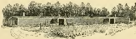
2404. A half-cellar storage.
