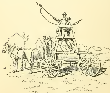
2378. Orchard pump with conical tower rig.
