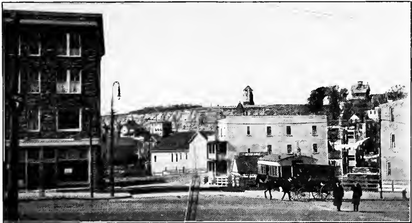
FIG. 13.—BREED'S HILL, FROM SARATOGA STREET BRIDGE.
