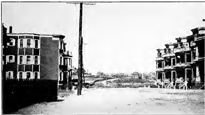
FIG. 45.—AUSTIN AVENUE, NORTH FROM SARATOGA STREET.
