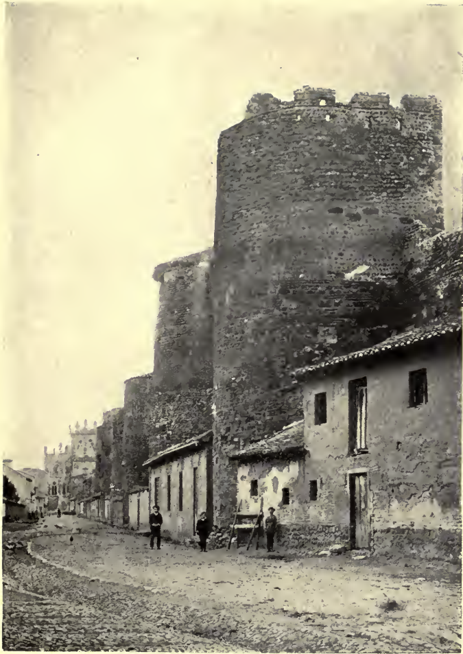
The Roman walls of Leon
