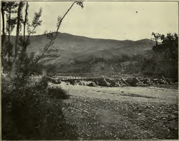
DAM ON THE RIVER GENIL, SPAIN.
