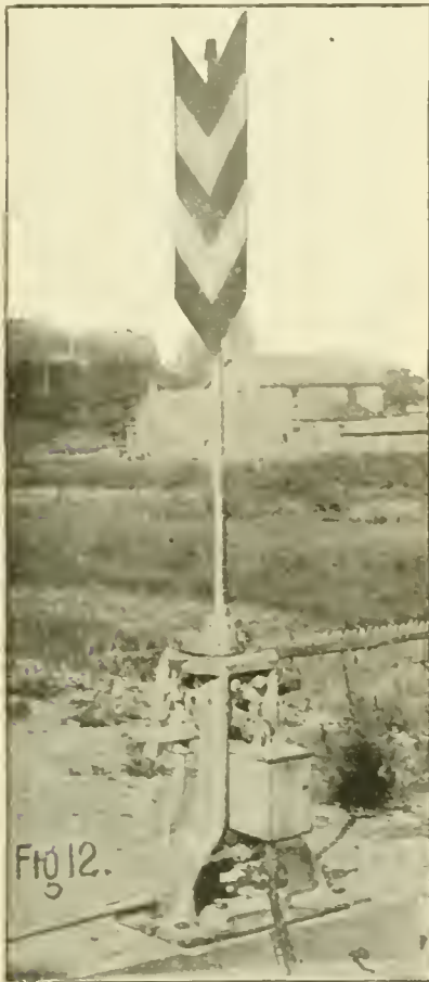
ELLIOTT'S ELECTRICALLY-LOCKED SWITCH STAND.
