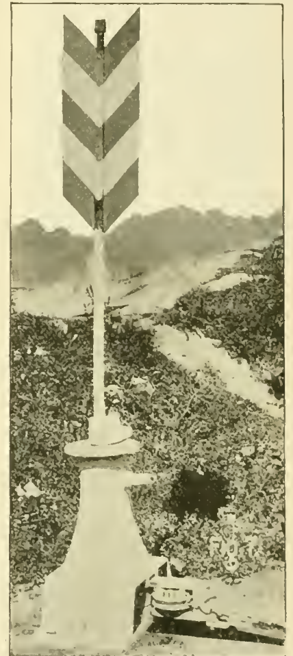
GIBBS' INTERLOCKING SWITCH STAND AT "DANGER."
