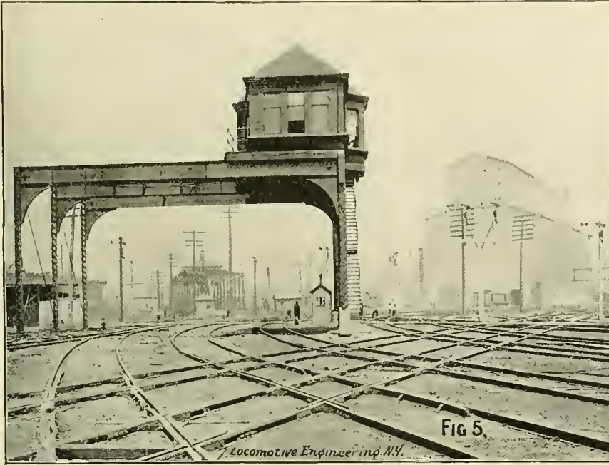
TOWER HOUSE FOR ELECTRO-PNEUMATIC.
