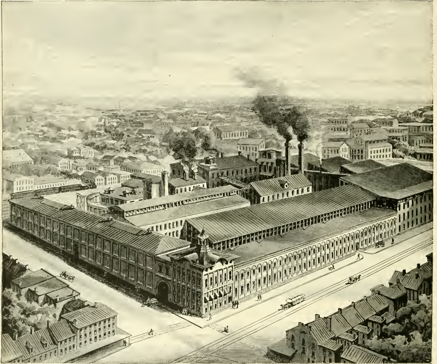
VIEW OF 21ST STREET WORKS.
