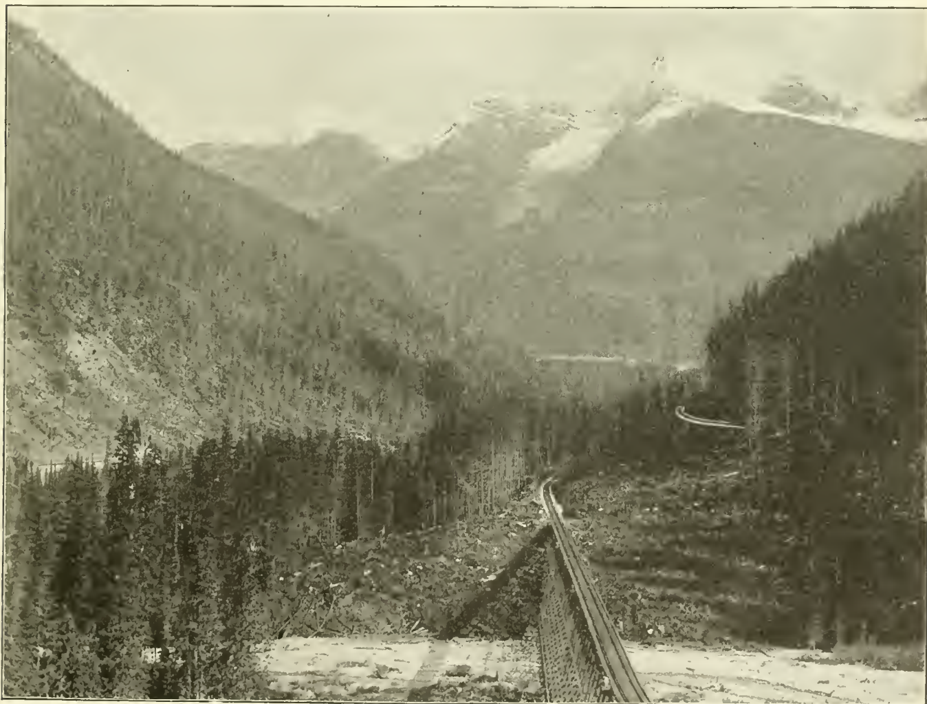
FOUR-TRACK VIEW, CANADIAN PACIFIC RAILROAD, SELKIRK MOUNTAINS.
