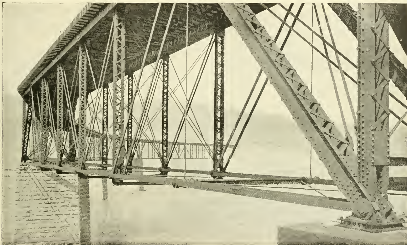
CURVED BRIDGE ON NORFOLK & WESTERN, NEAR PULASKI.
