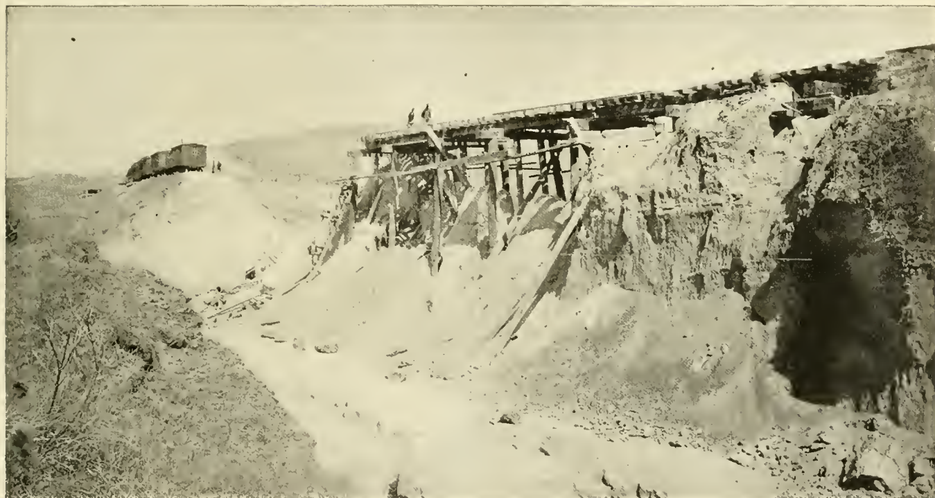
GREAT WASHOUT ON CHEYENNE & HOLDREGE BRANCH OF THE "BURLINGTON" LINE, APRIL 18, 1896. 350 FEET LONG, 65 FEET DEEP.
