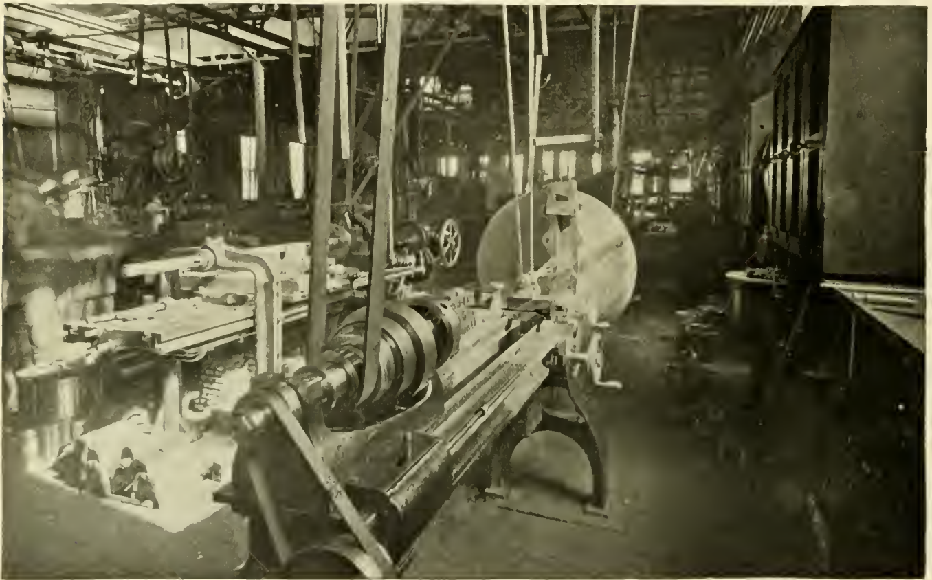
Fig. 1 EMERY WHEEL GRINDER FOR HARDENED BUSHES.
