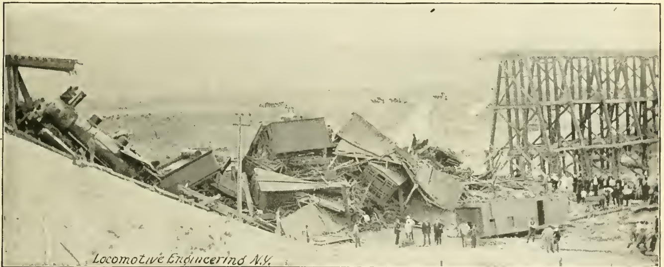
RESULT OF NOT SUPPORTING AN OLD BRIDGE WHILE PUTTING A NEW ONE UNDER IT.
