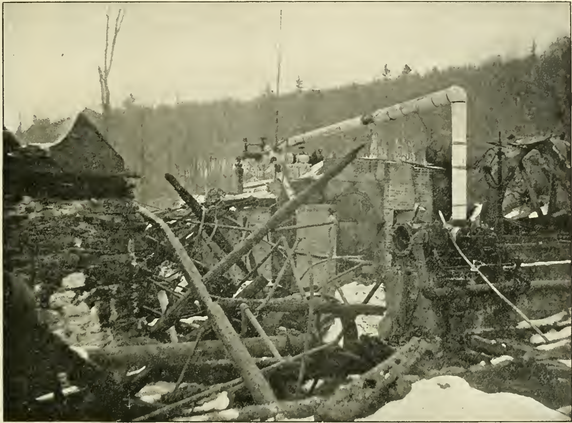
Ruins of the A. W. Eaton Paper Co.'s Mill, at Lee, Mass. SHOWING FIRE-PROOF CHARACTER OF THE MAGNESIA SECTIONAL COVERINGS.
