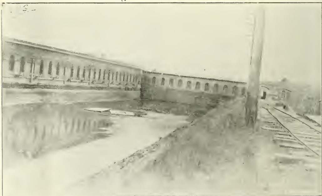
Power Canal.—Water low, showing source of water supply.—Sault Ste. Marie.
