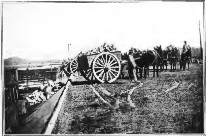
FIG. 8.—Caliche at the crusher.
