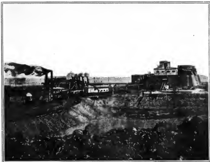
FIG. 10.—Machinery used in preparing the nitrate and iodine.
