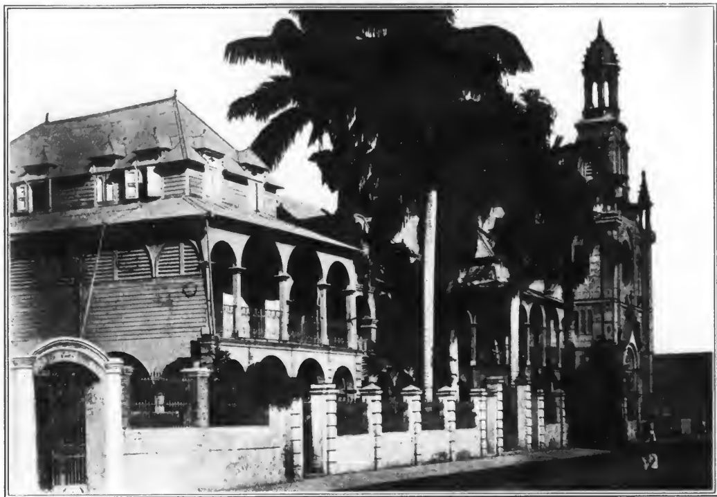
PRIMARY SCHOOL OF THE BROTHERS OF THE CHRISTIAN SCHOOLS, PORT AU PRINCE, HAITI.
