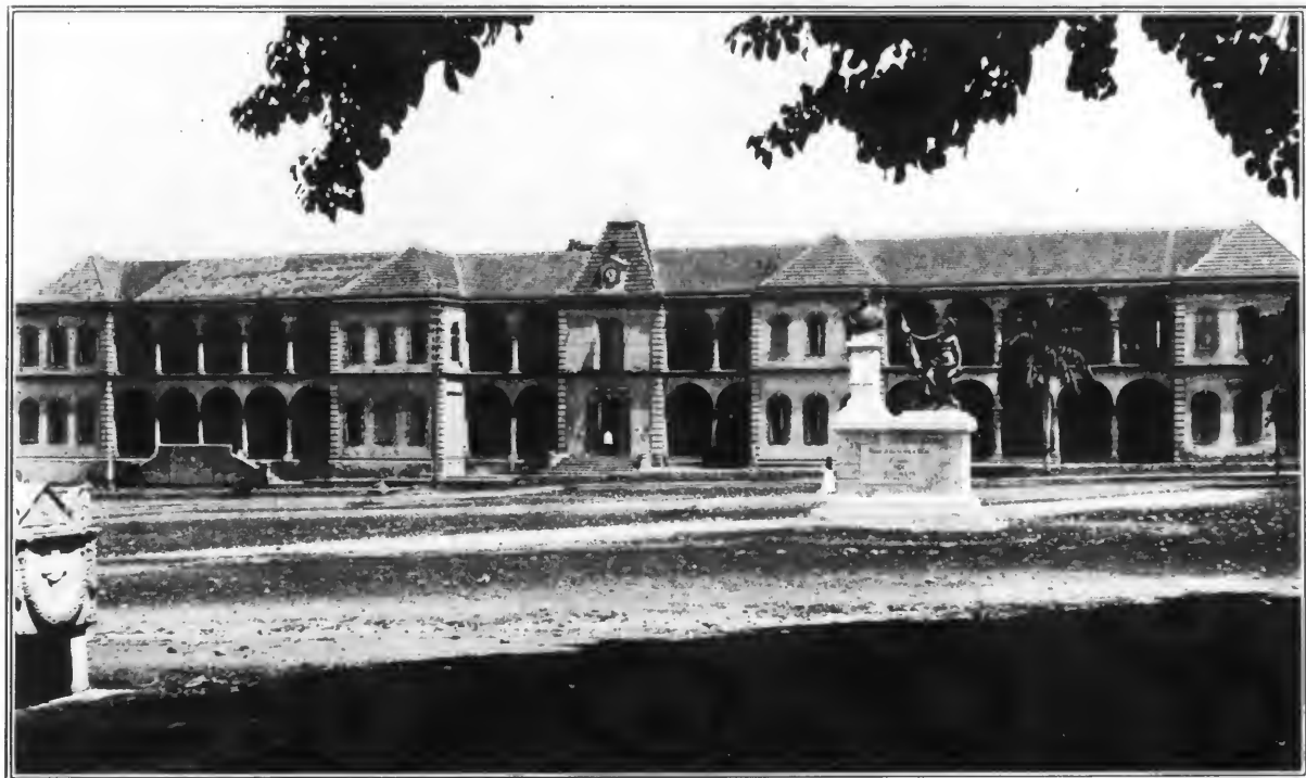
GOVERNMENT BUILDING, PORT AU PRINCE, HAITI.
