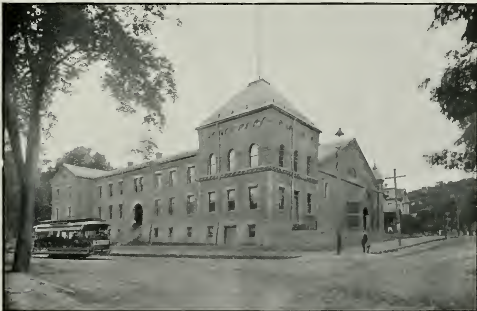
THE ARMORY—COIT AND WASHINGTON STREETS.
