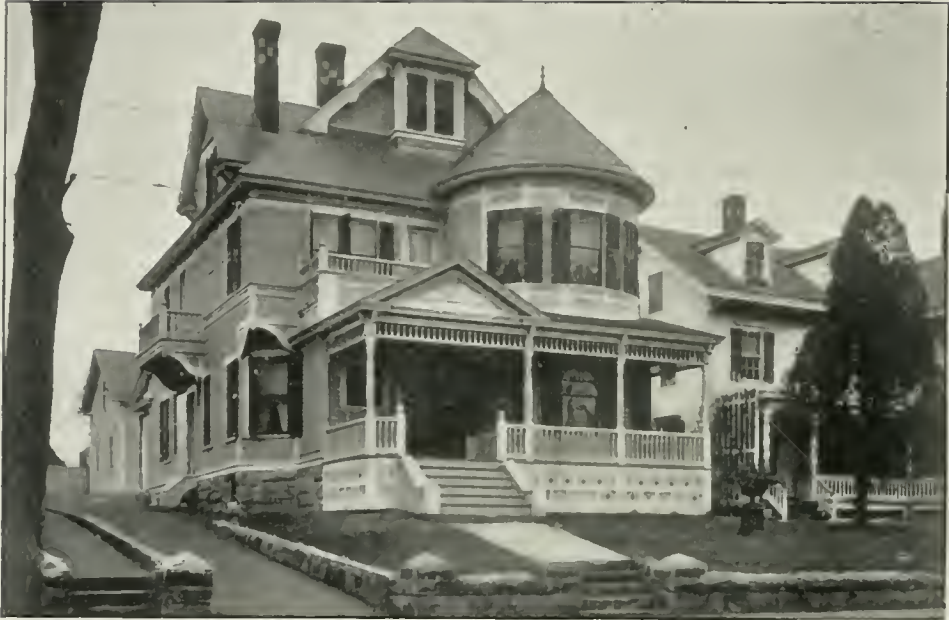
RESIDENCE OF JOHN B. LEAHY—4 CHANNING STREET.
