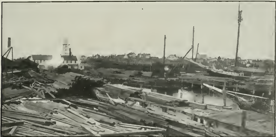
VIEW IN THE ROBERT PALMER & SON SHIPBUILDING AND MARINE RAIL- WAY COMPANY'S YARD—SHOWING WORK UNDER CONSTRUCTION AND VESSELS ON THE WAYS.
