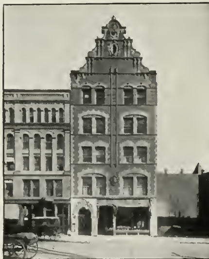
OFFICE OF THE N. E. ENGINEERING CO. Waterbury, Connecticut.
