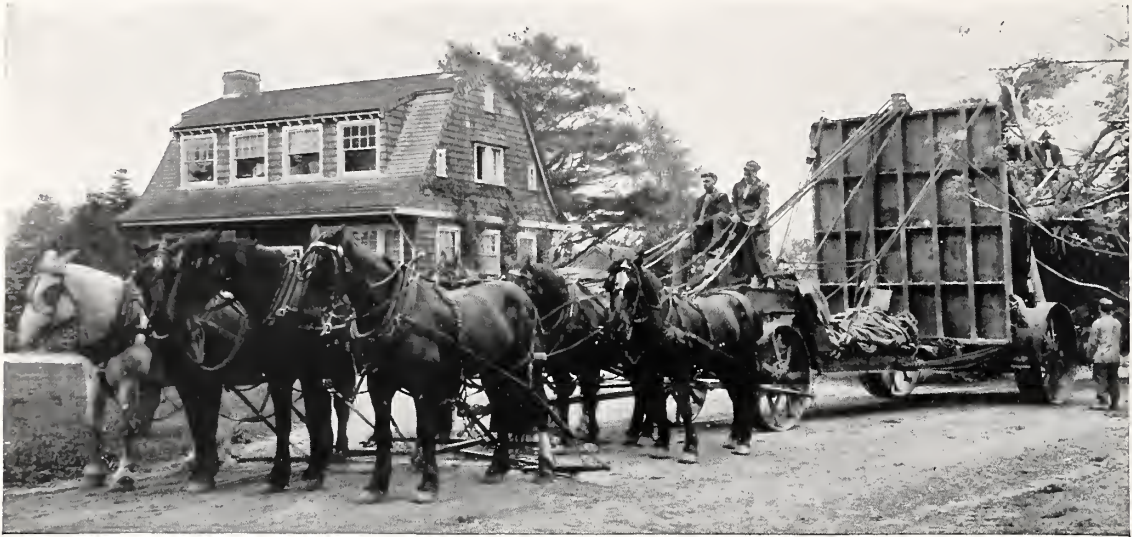
Tree-Mover No. 21. Moves evergreens and other trees with very large balls of earth. This is one of two Pines moved from our nursery to the church half a mile east. The big steel platform and frame are worth seeing
