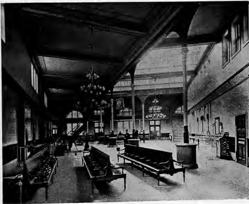
INTERIOR OF LONG ISLAND RAILROAD STATION, FLATBUSH AVENUE.
