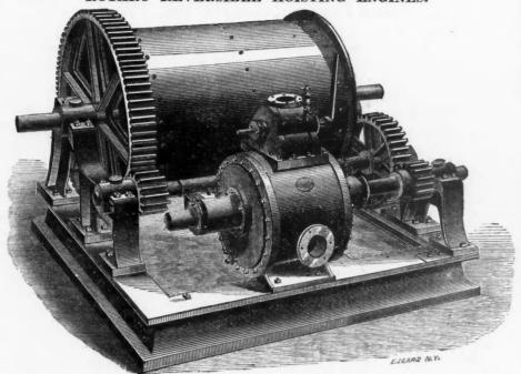
We can refer to the satisfactory performance, during the last tirree years, of over TWO HUNDRED of these Engines, from the little Ash Hoister on steamships, raising 300 pounds, to the Mining and Quarrying Engines, laising 6,000 to 60 000 lb. These Engines have no dead centres; one lever raises, lowers, and holds the load; are simple, cheap, durable, effective.
