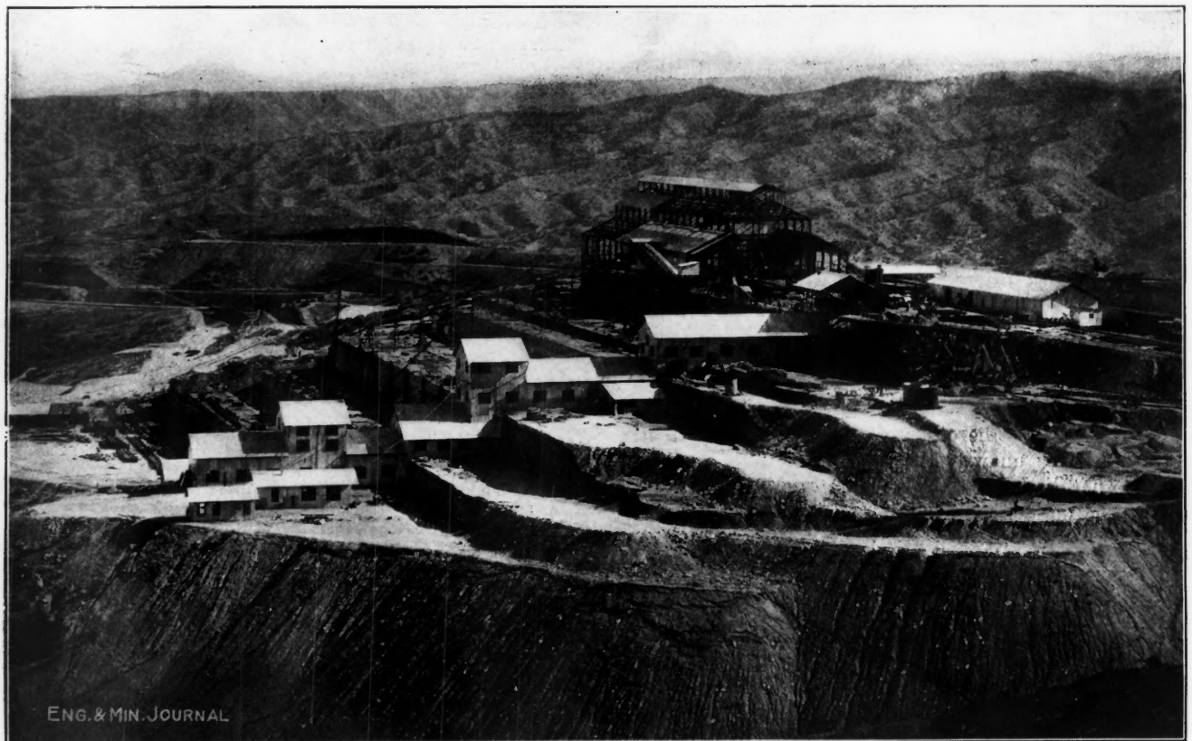
INSPIRATION CONSOLIDATED 8000-TON MILL NOW BEING BUILT
