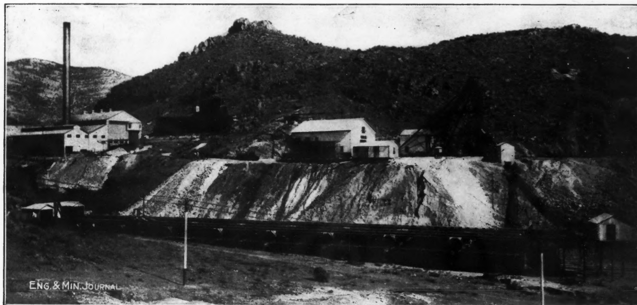
Copper Queen main power house
