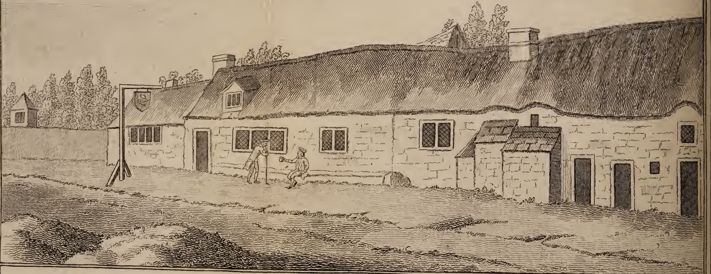
The Revolution House at Whittington near Chesterfield, Derbyshire.
