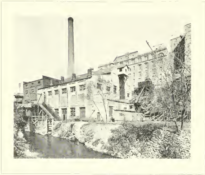
"A" Mill Power House
