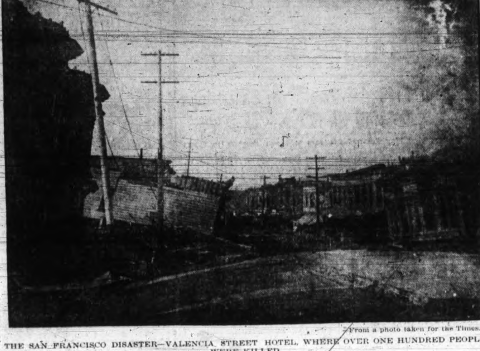
THE SAN FRANCISCO DISASTER—VALENCIA STREET HOTEL, WHERE OVER ONE HUNDRED PEOPLE WERE KILLED.
