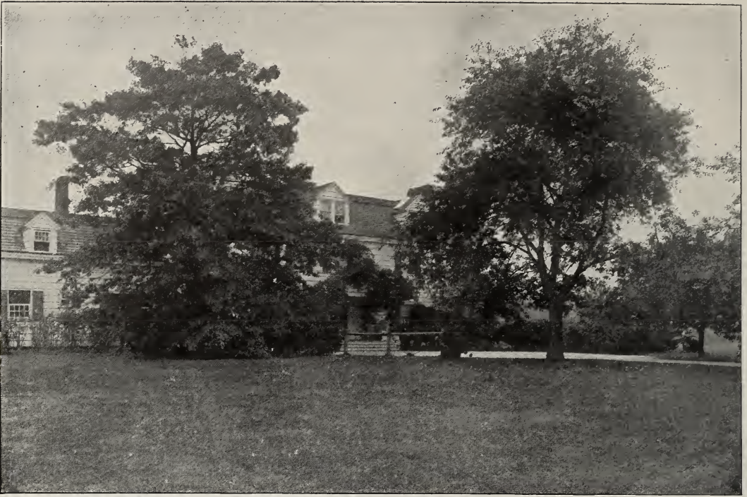
Permanent success results from moving trees with Hicks' Patent Tree-Movers. This Pin Oak and Wild Cherry were moved in 1897, and photograph taken 1905. They grow at the full normal rate. Residence of John L. Lawrence, Lawrence, L. I.
