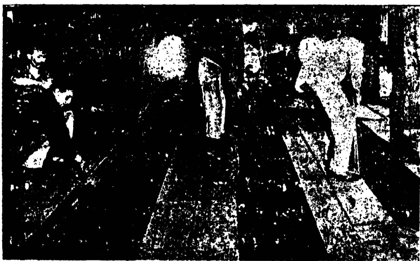
BLOWING WINDOW GLASS CYLINDERS BY HAND.
