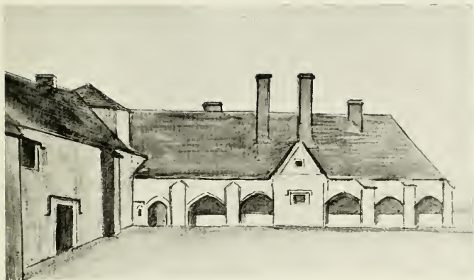
REMAINS OF LORD LUMLEY'S HOUSE AT STANSIEAD
