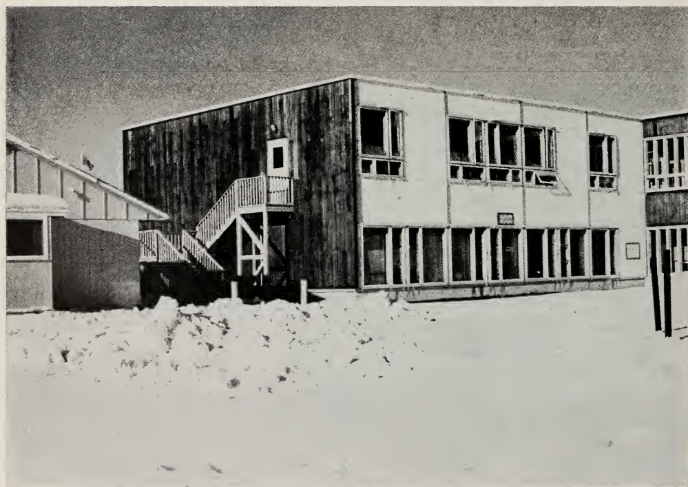
Dining and Recreation Hall — Ontario Reformatory, Elliot Lake
