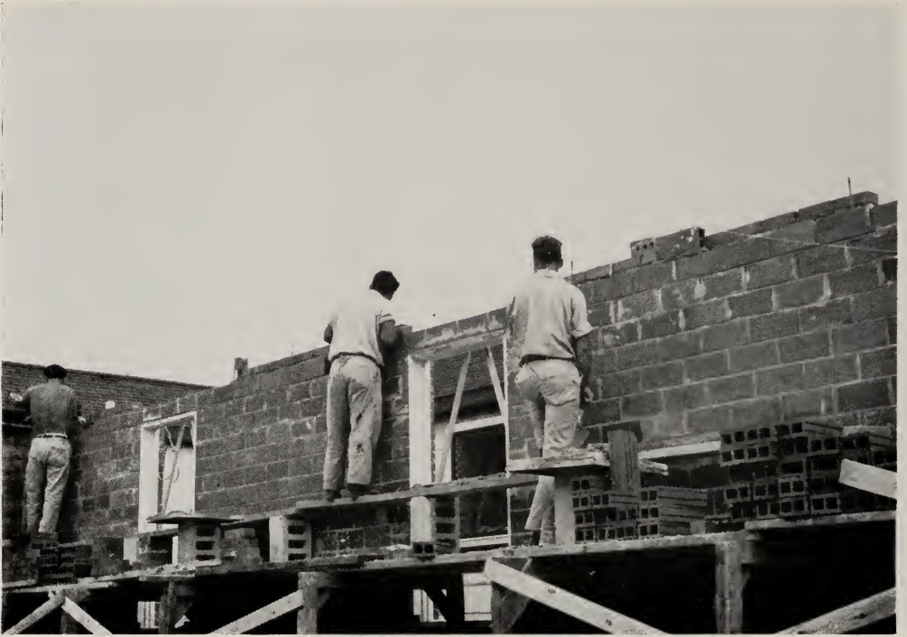
Chapel under construction — Burtch Industrial Farm, Brantford.
