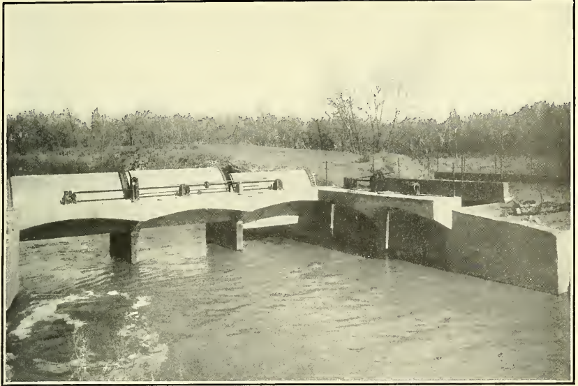
FIG. 1.—SAND AND WASTE GATE, AMITY CANAL, COLORADO.
