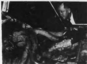
FAA GENERAL SAFETY INSPECTOR examines the engine of a large transport after it has received a periodic overhaul. All work on general aviation aircraft and engines is thoroughly inspected by these men.
