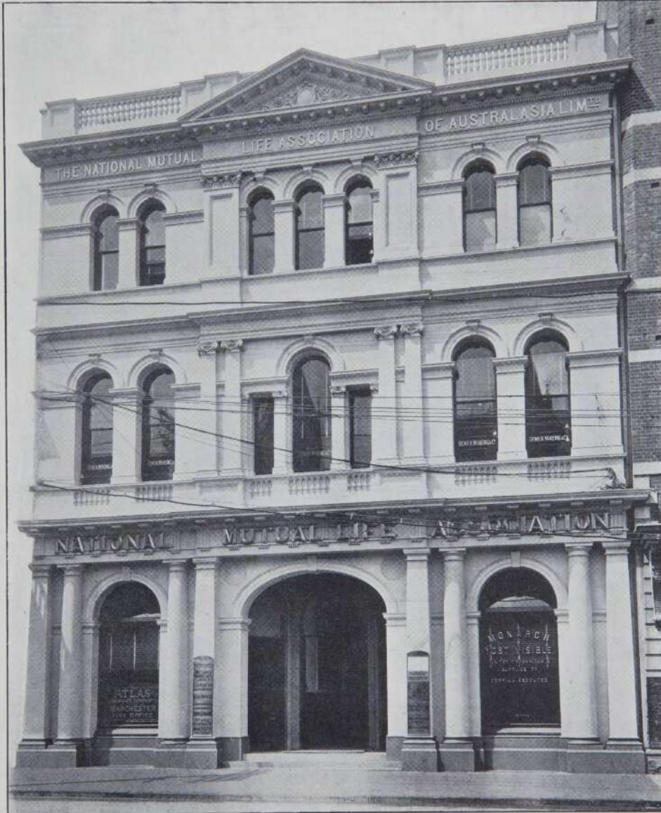
OFFICES OF THE NATIONAL MUTUAL LIFE ASSOCIATION, ST. GEORGE'S TERRACE, PERTH.
