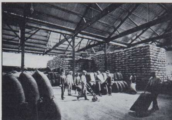
Photo by C. E. Farr. INTERIOR VIEW OF NO. 1 SHED, SHOWING FLOUR STACKS, "PEERLESS" ROLLER FLOUR MILLS
