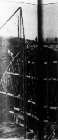
FIG. 3.—VIEW OF FALSEWORK
