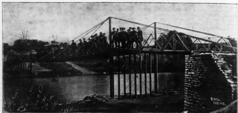
FIG. 2.—MITCHELL STEEL CABLE BRIDGE OVER WHITWATER RIVER, AT RICHMOND, IND. Built by Mitchell Bridge Co., 1889. Washed away, 1897.
