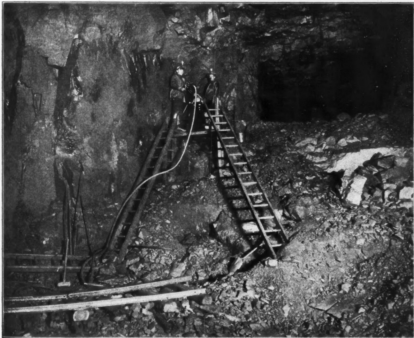
FIG. 1. UNDERHAND BENCH STOPE IN CLEVELAND CLIFFS IRON CO. MINE
