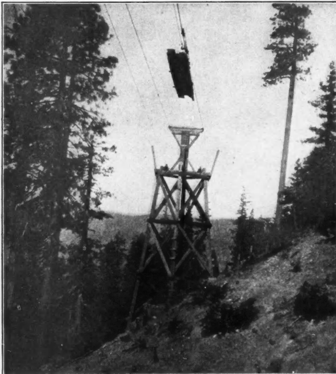
FIG. 1. LOAD OF LUMBER ON TRAMWAY NEAR QUINCY, PLUMAS COUNTY, CALIF.
