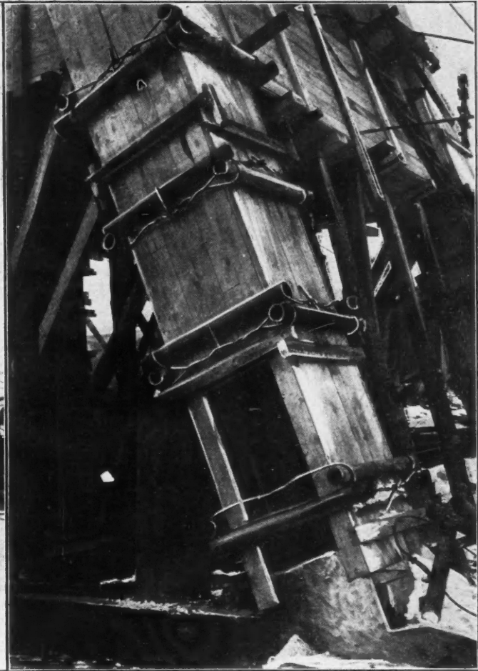
COLUMN-FORM YOKES OF SCRAP BOILER FLUES AND SCRAP 1/2-IN. STEEL ROPE
