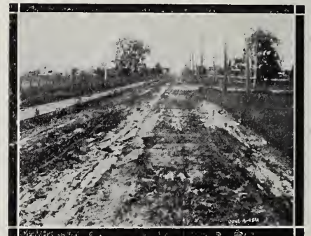
A typical mud hole before improvement
