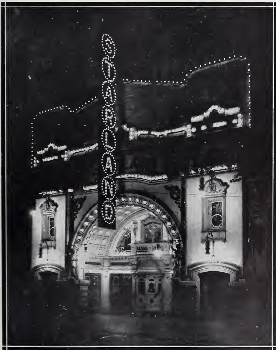
Exterior View of Starland Building by night
