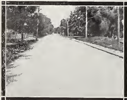
A concrete country road
