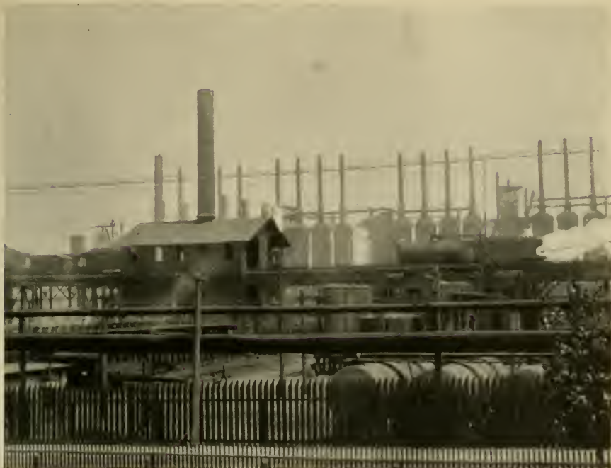
FIG. 1.—VIEW OF MODERN BY-PRODUCT COKE-OVEN PLANT WITH IRON FURNACE IN BACKGROUND.
