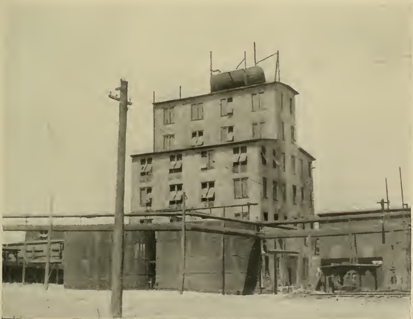
FIG. 2.—BY-PRODUCT HOUSE CONTAINING AMMONIA STILLS.
