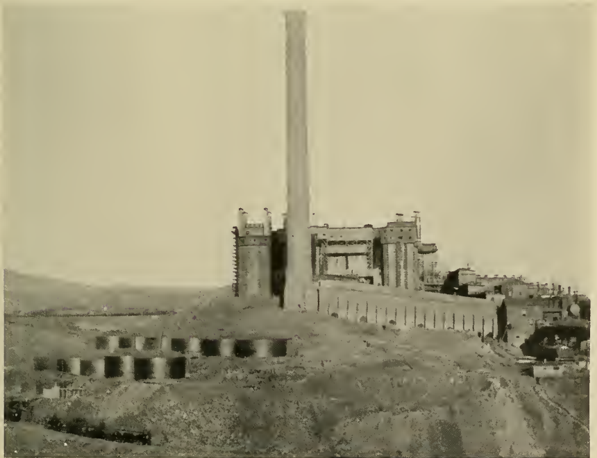
FIG. 2.—SIDE VIEW OF SAME PLANT, SHOWING STORAGE TANKS FOR ACID.
