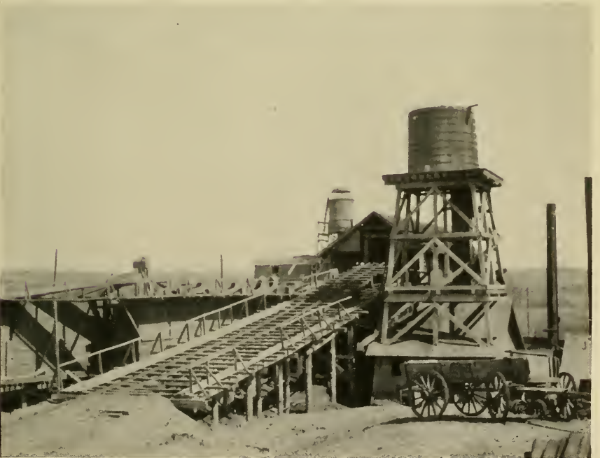
FIG. 2.—ANOTHER VIEW OF THE SAME PLANT, SHOWING HOOD OVER STACK AND SETTLING TANKS FOR FINELY DIVIDED PHOSPHATE.
