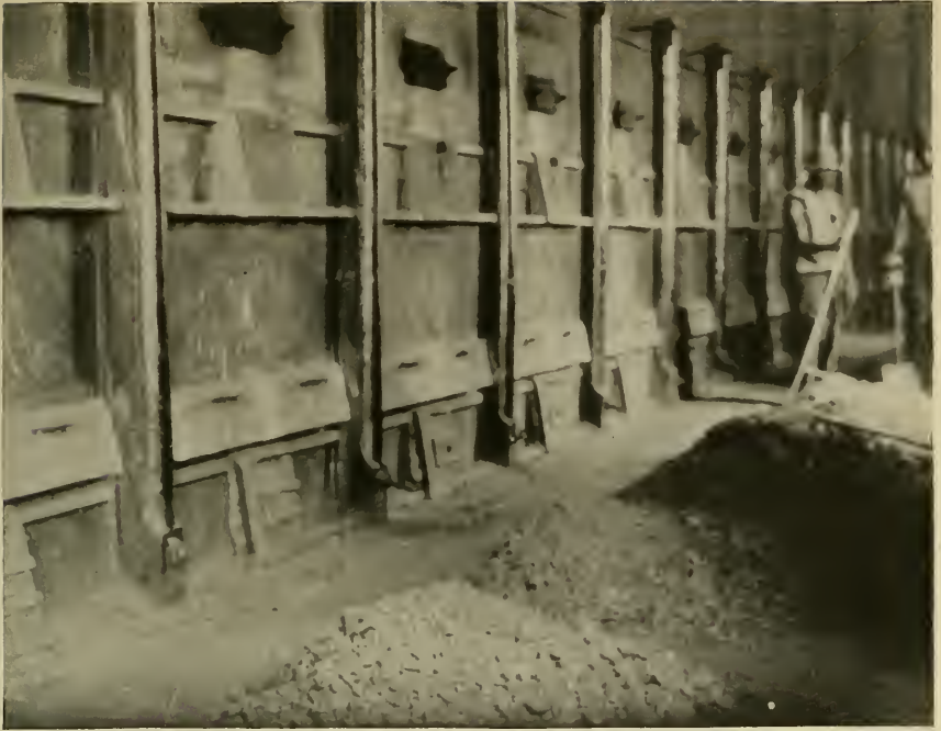
FIG. 1.—BATTERY OF PYRITES BURNERS.
