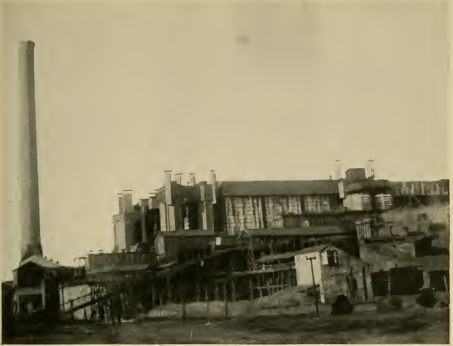
FIG. 1.—FRONT VIEW OF ACID PLANT RUN IN CONNECTION WITH A COPPER MINE.
