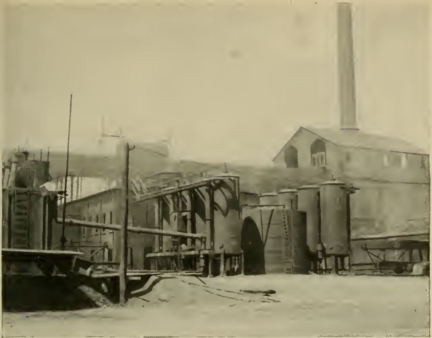
FIG. 1.—VIEW OF TAR AND LIQUOR CONDENSERS.
