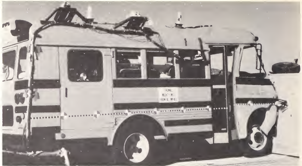
Crash protection systems for wheelchair occupants are being tested jointly with the National Highway Safety Administration's schoolbus test program.
