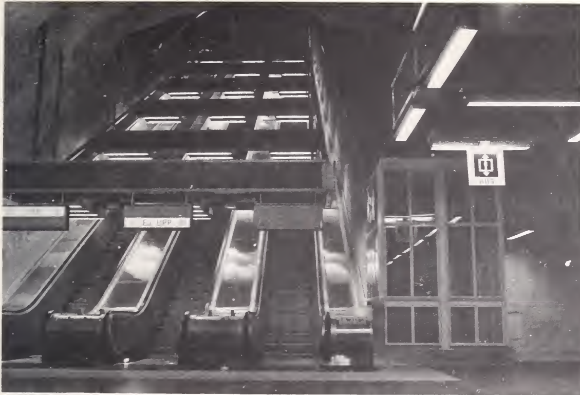
Elevators which parallel the incline of neighboring escalators accommodate wheelchair users in the Stockholm subway. The elevator has direct access to the sidewalk with no intervening architectural barriers.
