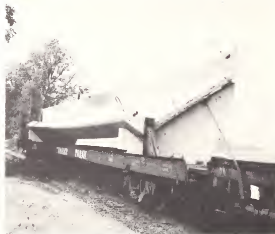
The use of prefabricated guideway sections is being evaluated under the AGT Supporting Technology Program.
