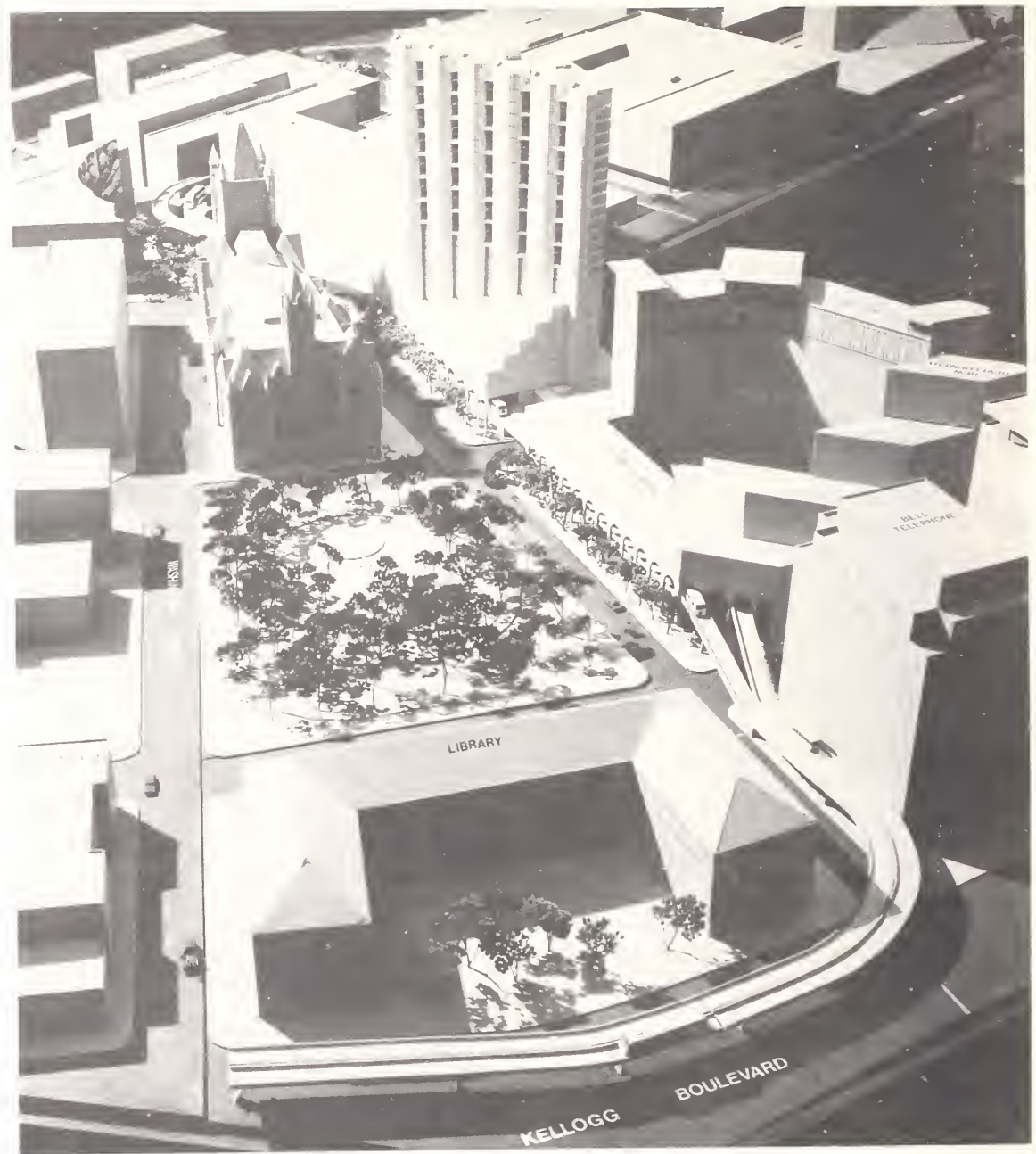
This architectural model shows a preliminary DPM design for St. Paul, Minn. Here, the DPM enters and makes a loop through a proposed new building complex.
