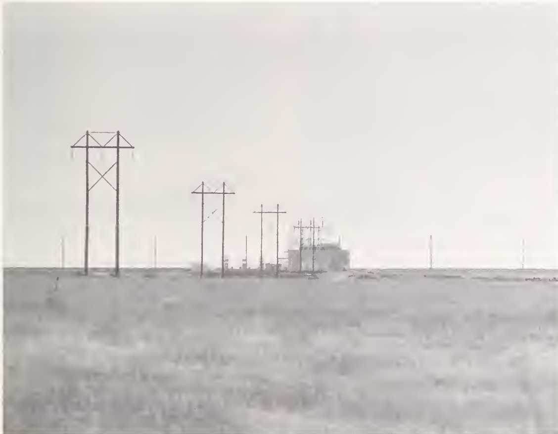
Power substations have been constructed at the Transportation Test Center to supply electricity for rail car testing. Pike's Peak is in the background.
