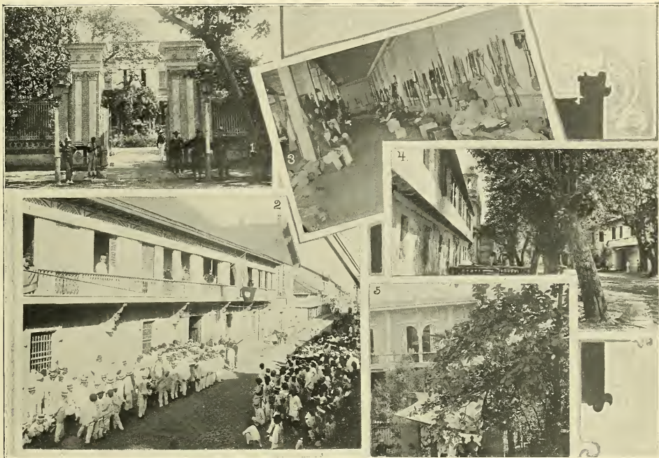
1—General McArthur's headquarters, San Miguel. 2—Filipinos obtaining identification certificates at Kansas headquarters. 3—Interior of army barracks. 4—The oldest church in the Islands and first headquarters of Aguinaldo, Cavite. 5—South Dakota headquarters.
