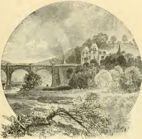
VIADUCT AT RELAY.
