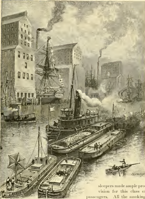
LOCUST POINT — ELEVATORS.
