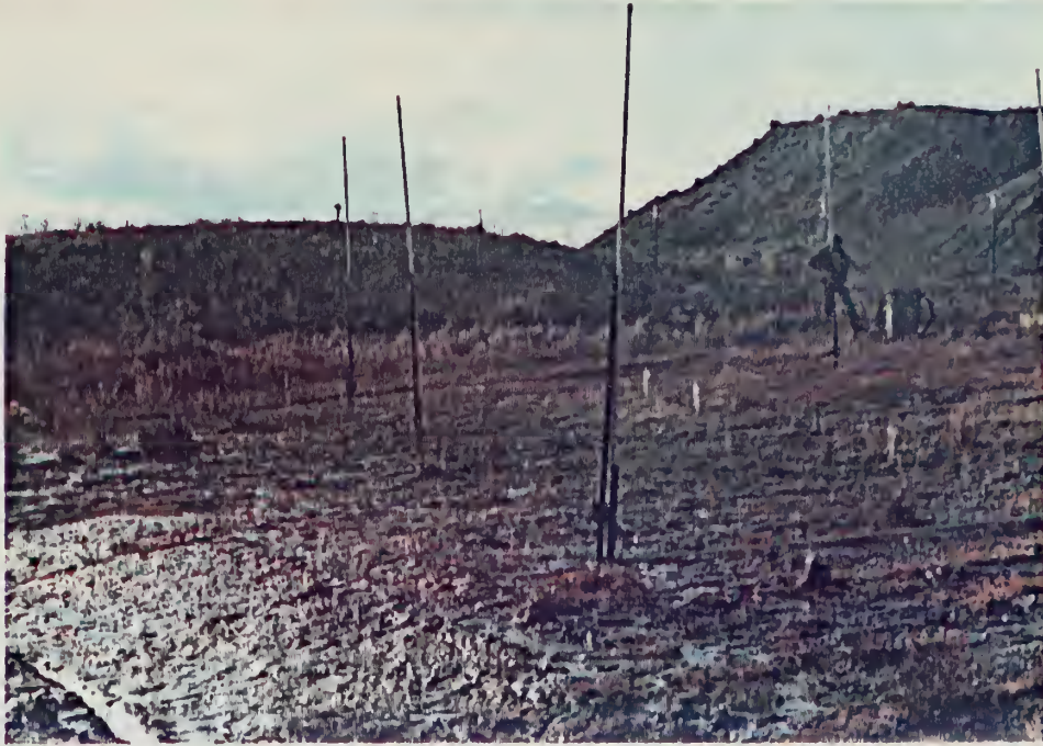
Onset of Puddling - Runoff
