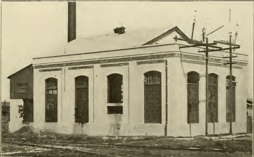
New electric plant at Caibarien.
