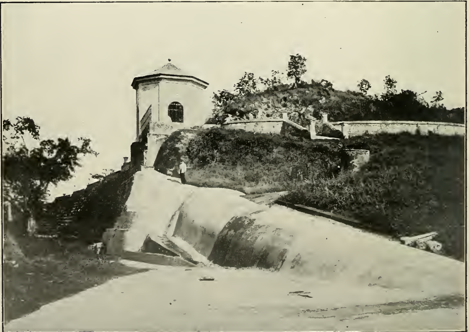
The tunnels which convey the water from the Vento springs to Havana
