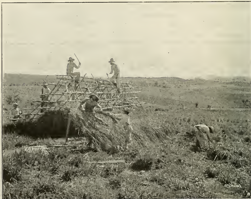
Beginnings of a Cuban home
