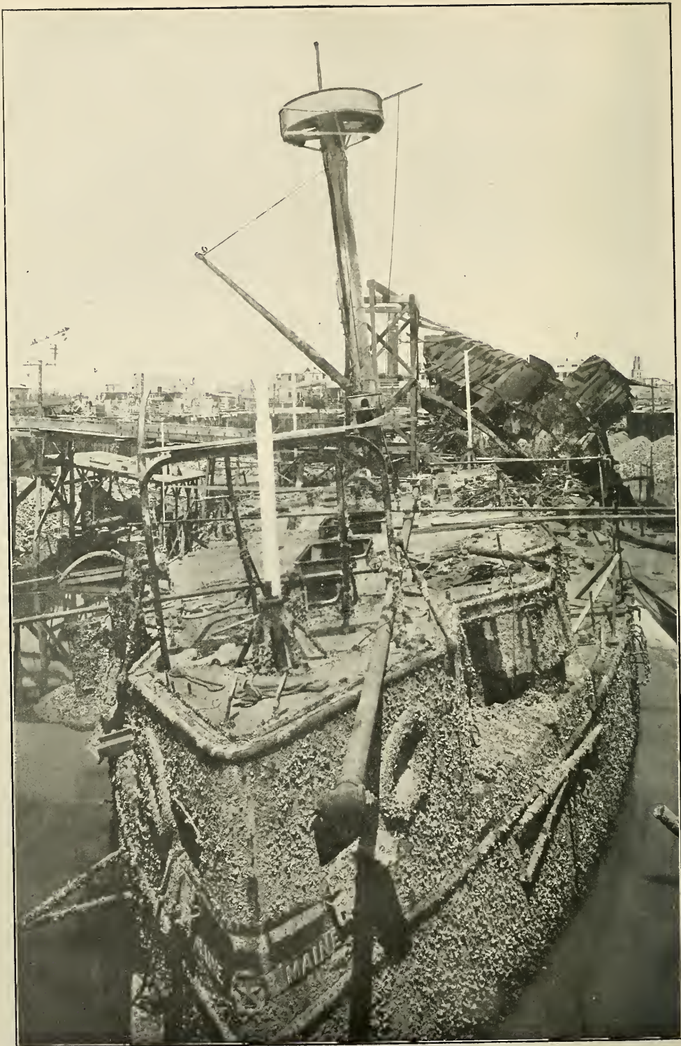
The battleship "Maine" within the cofferdam. The sea of mud which still surrounds her is 25 feet deep. The encrustations appearing on the hull are all oysters and barnacles.
