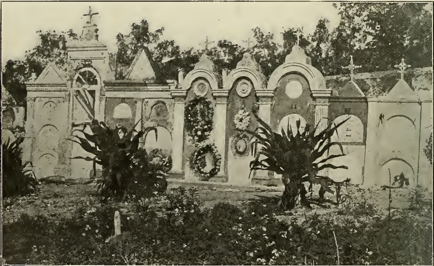
Cemetery at Nuevitas. The vaults are above ground and the semi-circular opening after interment is sealed with cement. A mortuary tablet is then placed on the cement surface.
