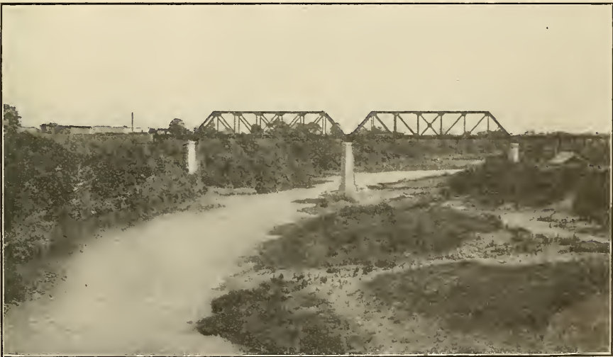
New Cuba Railroad bridges in Cuba. They cross the Bayamo River.
