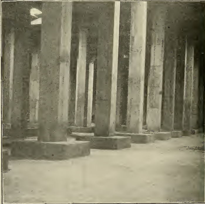
Interior of the reservoir, showing the pillars which support the roof.
