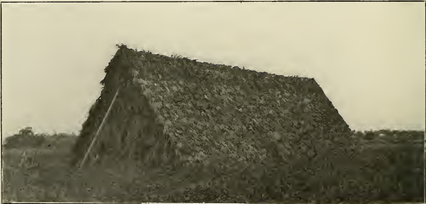
Old style of native curing shed, built almost entirely of palm leaves. A frame work of poles is first constructed, to which the long leaves of the royal palm are lashed and interwoven, making a watertight roof which, aside from loss by fire, will last for twenty or thirty years.
