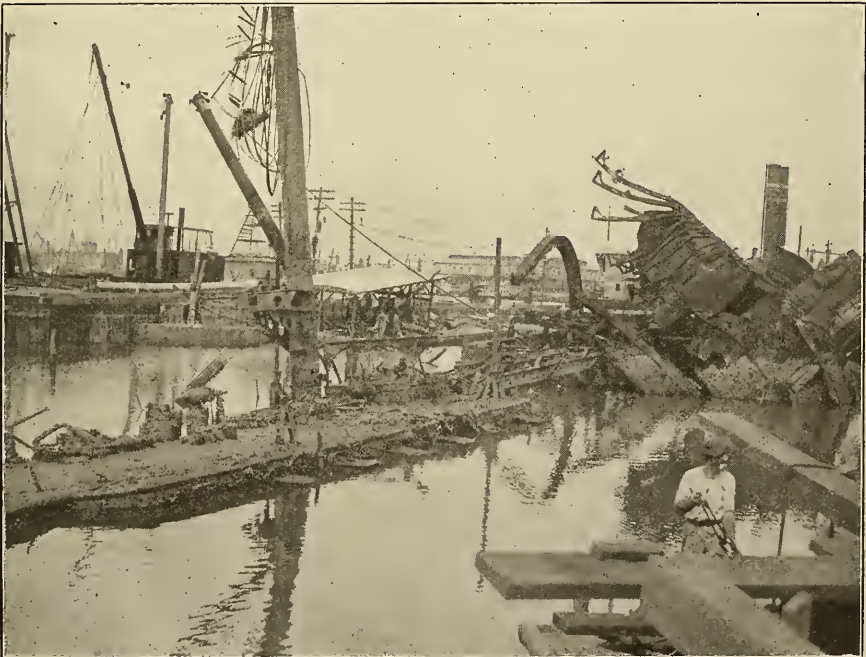
Photograph showing the "Maine" after the first pumping when the water within the cofferdam was lowered five feet. Note the barnacles and marine growth along the exposed decks. (Photo by Harris Bros., Havana.)
