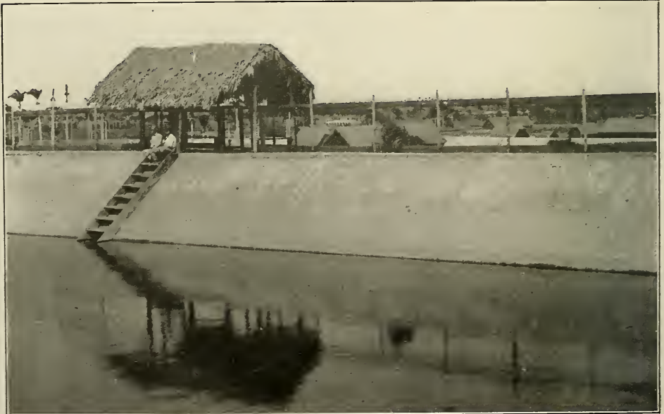
Reservoir at American Tobacco Co.'s plantation at Rio Seco. Part of the irrigation system, water for which is pumped from a stream some two miles distant.
