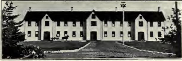
Calgary Barracks, erected in 1888-89.
