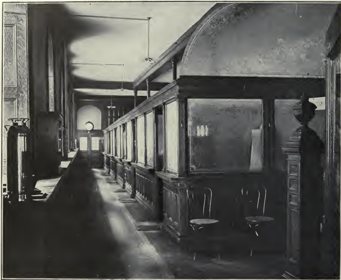
Interior View of Montreal Office.
