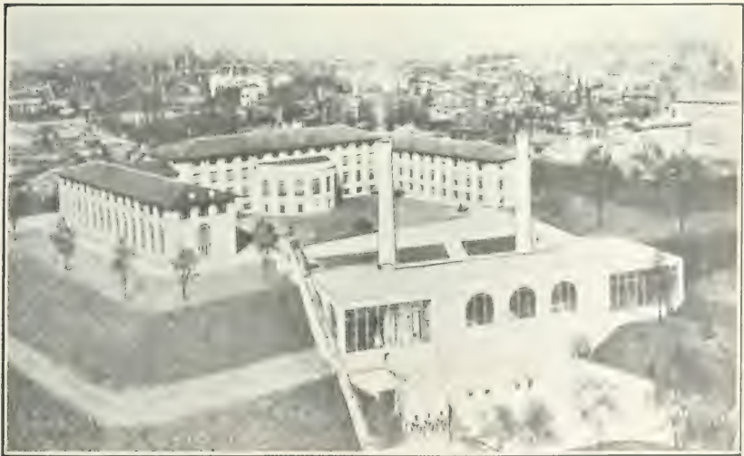
THE PITTSBURGH STATION FROM THE REAR.
