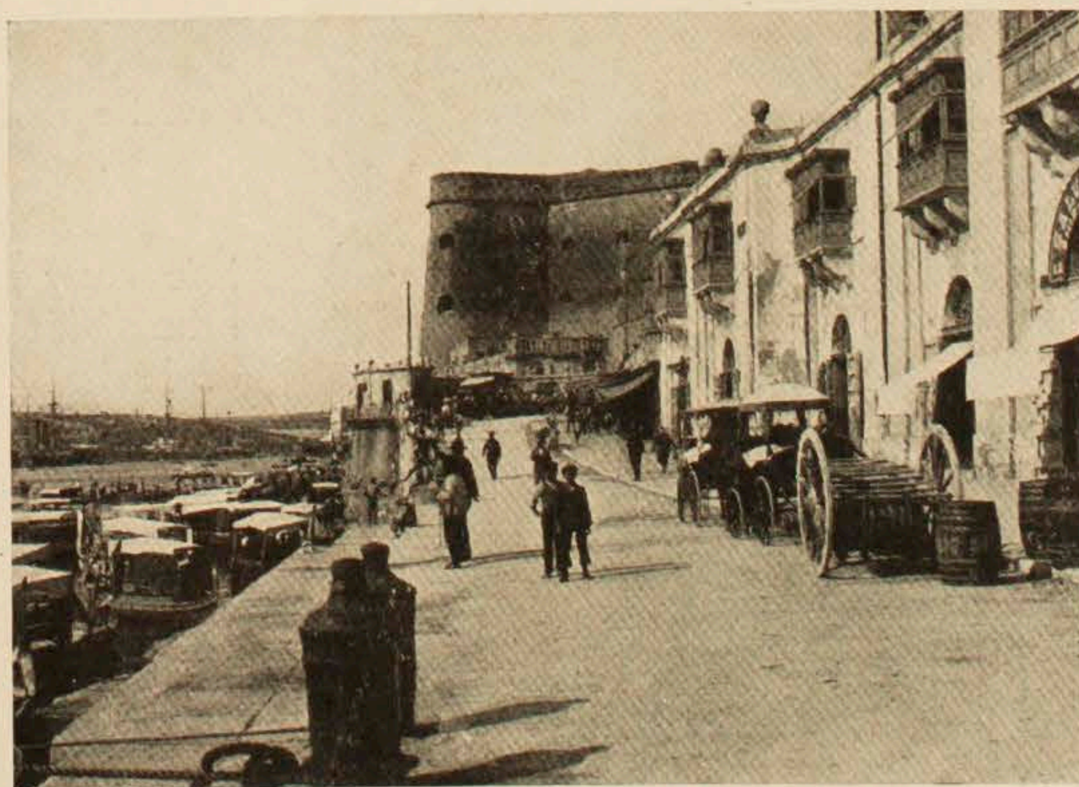
The waterfront at Valetta showing old cannon now used as mooring posts
