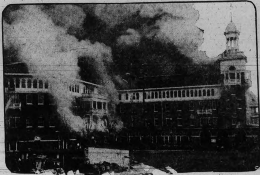
Firemen battling to save the Arlington Hotel, Hot Springs, Ark. They were unsuccessful and the structure was leveled after the fire had burned 10 hours, killing one and inflicting loss of $1,500,000.
