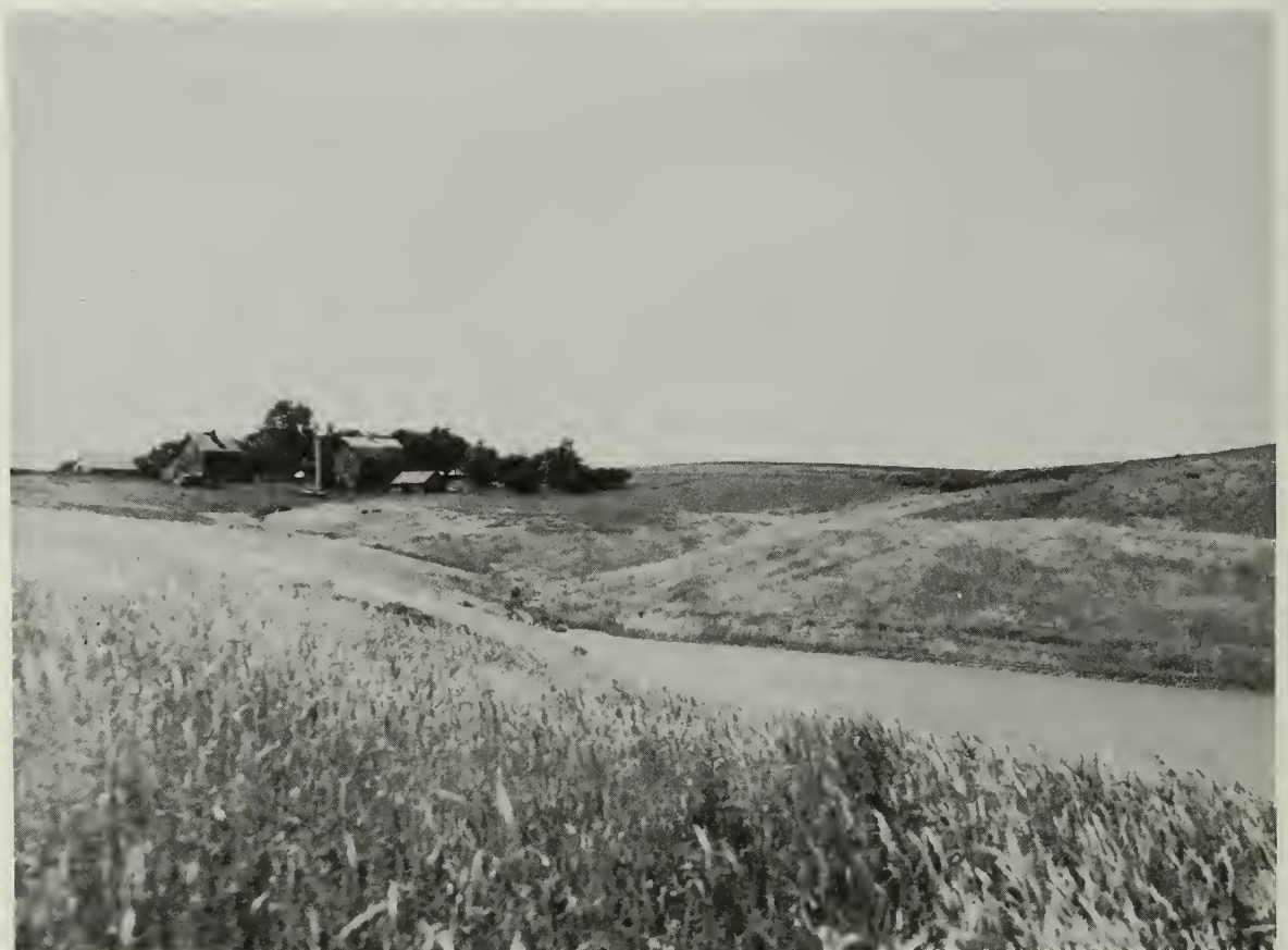
AFTER - SAME GULLY CONTROLLED BY STRUCTURE AND BY SHAPING AND SEEDING, ABOVE STRUCTURE.
