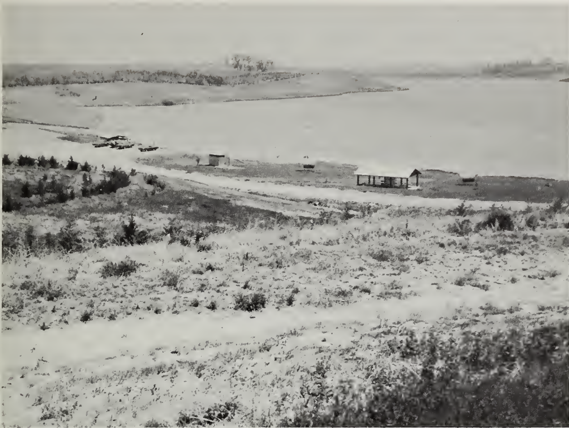
MORE OF THESE MULTIPURPOSE RECREATION AND FLOOD PREVENTION RESERVOIRS ARE NEEDED THROUGHOUT THE STUDY AREA.
