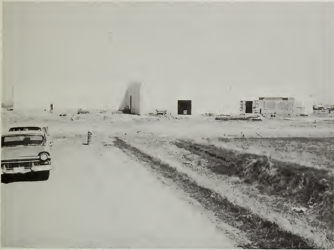
NEW 3-M PLANT BEING COMPLETED AT BROOKINGS, SOUTH DAKOTA.
