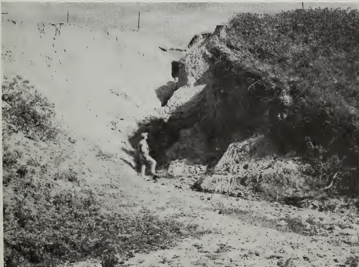
RUNOFF FROM ONLY 15 ACRES CAUSED THIS DEEP SCAR IN THE LANDSCAPE.
