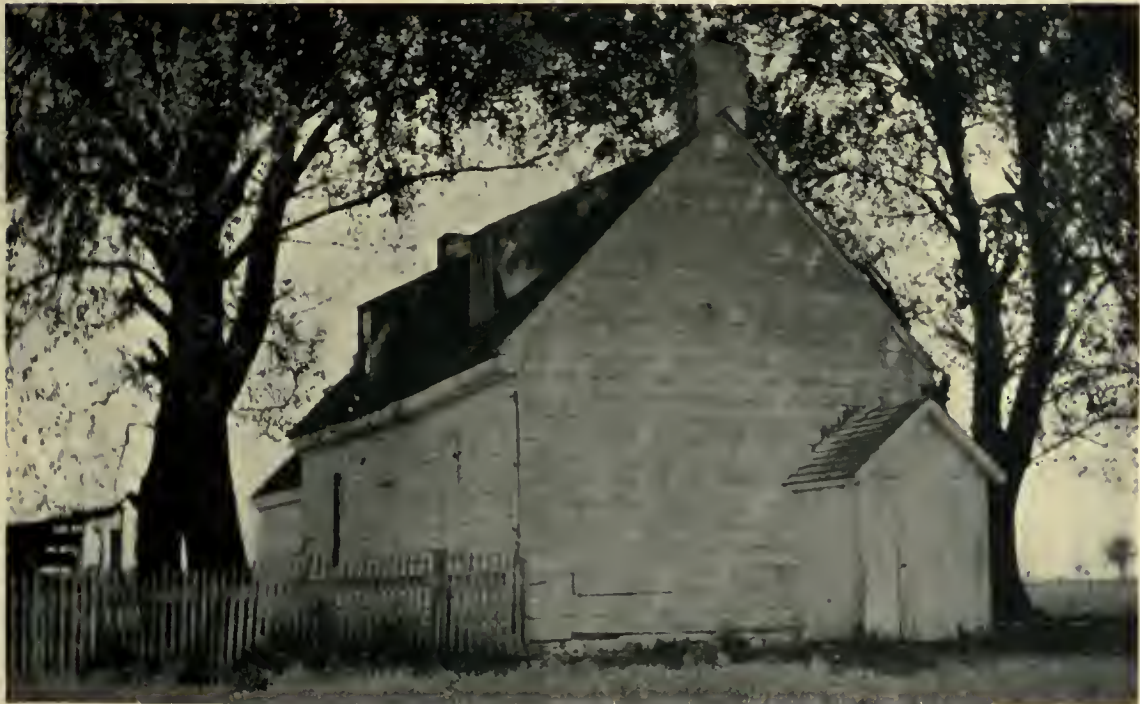
EARLY FARM-HOUSE ON MARYLAND STATE ROAD.
