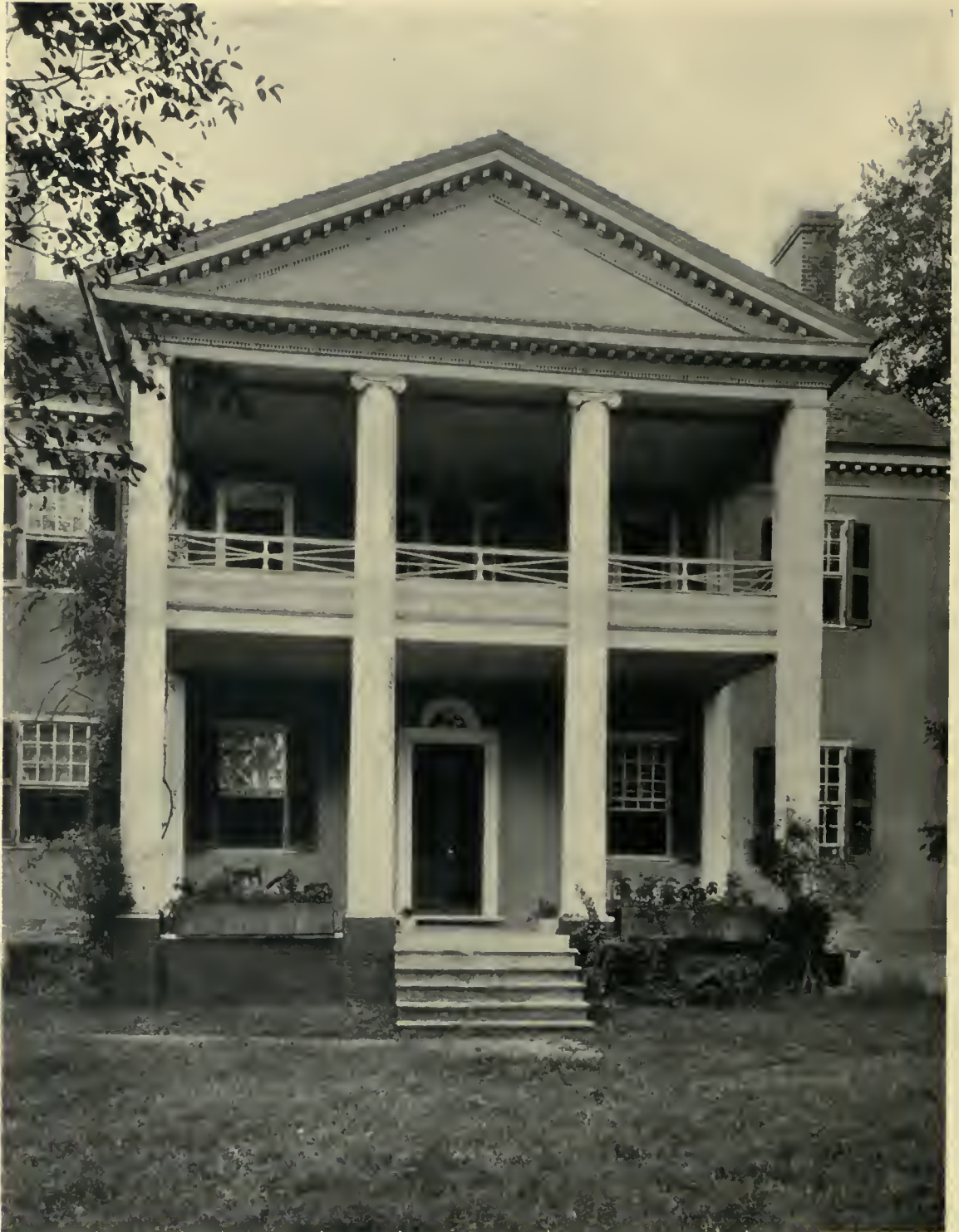
"BEVERLY" ON THE POCOMOKE RIVER, MARYLAND. Detail of Porch.
