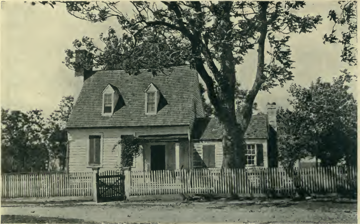
AN EARLY COTTAGE, FALMOUTH, VIRGINIA Long dormers with sharp-peaked gables are characteristic of the early Southern houses
