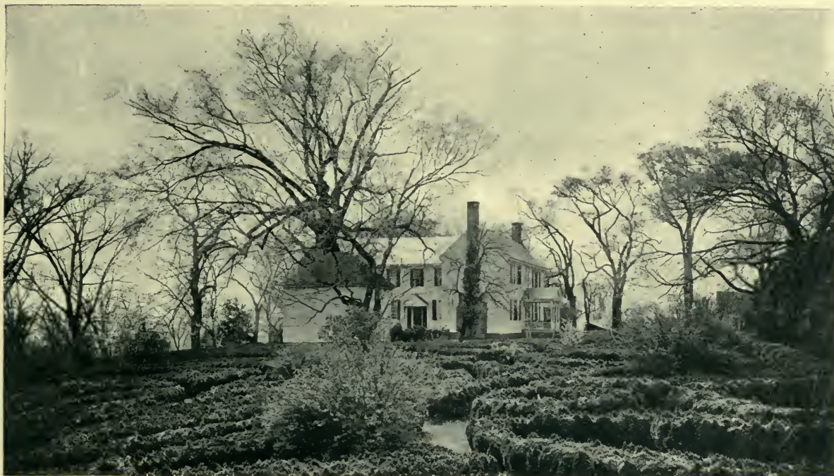
"TUCKAHOE," GOOCHLAND COUNTY, VIRGINIA. Built about 1707
