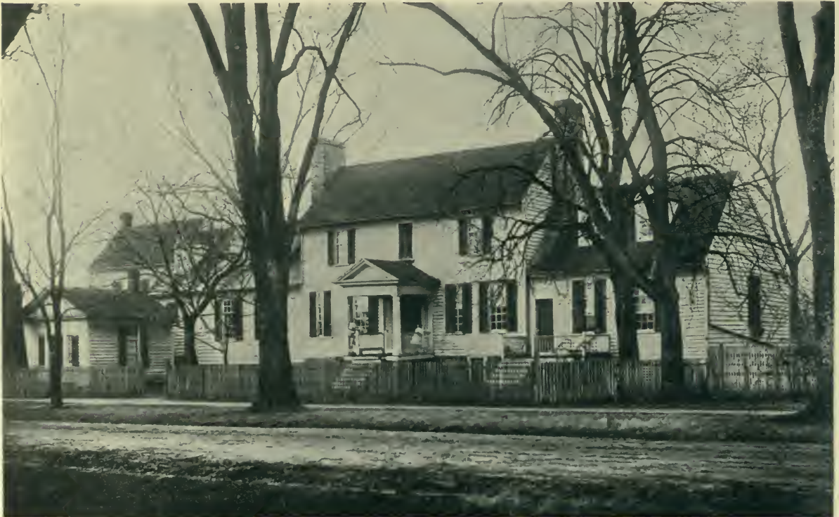
TUCKER HOUSE, WILLIAMSBURG, VIRGINIA The houses in this section followed the same general plan, the various departments located in ells or extensions clustered in a rambling manner about the central building. This house, like a majority of the Southern Colonial houses, has a bedroom on the ground floor. The windows are glazed with small panes set in lead
