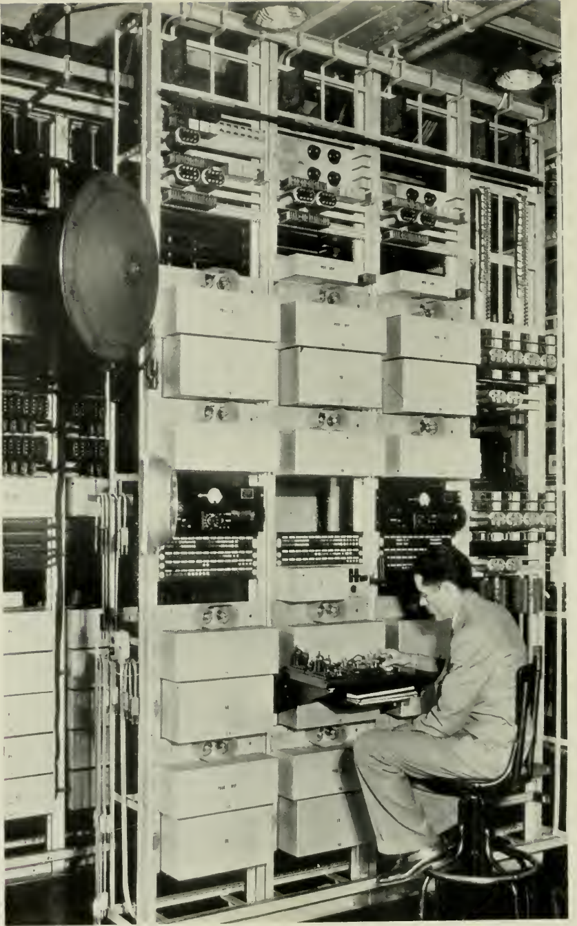
FIGURE 6. IN THE COURSE OF ITS JOURNEY ALONG WIRES, A RADIO PROGRAM PASSES THROUGH NUMEROUS TELEPHONE COMPANY "REPEATER" STATIONS. HERE, AS THE TERM SUGGESTS, THE WEAKENED CURRENTS ARE AMPLIFIED TO THEIR ORIGINAL STRENGTH AND QUALITY, AND ARE SENT ALONG TO THE NEXT SUCH STATION, WHERE THE PROCESS IS REPEATED.
