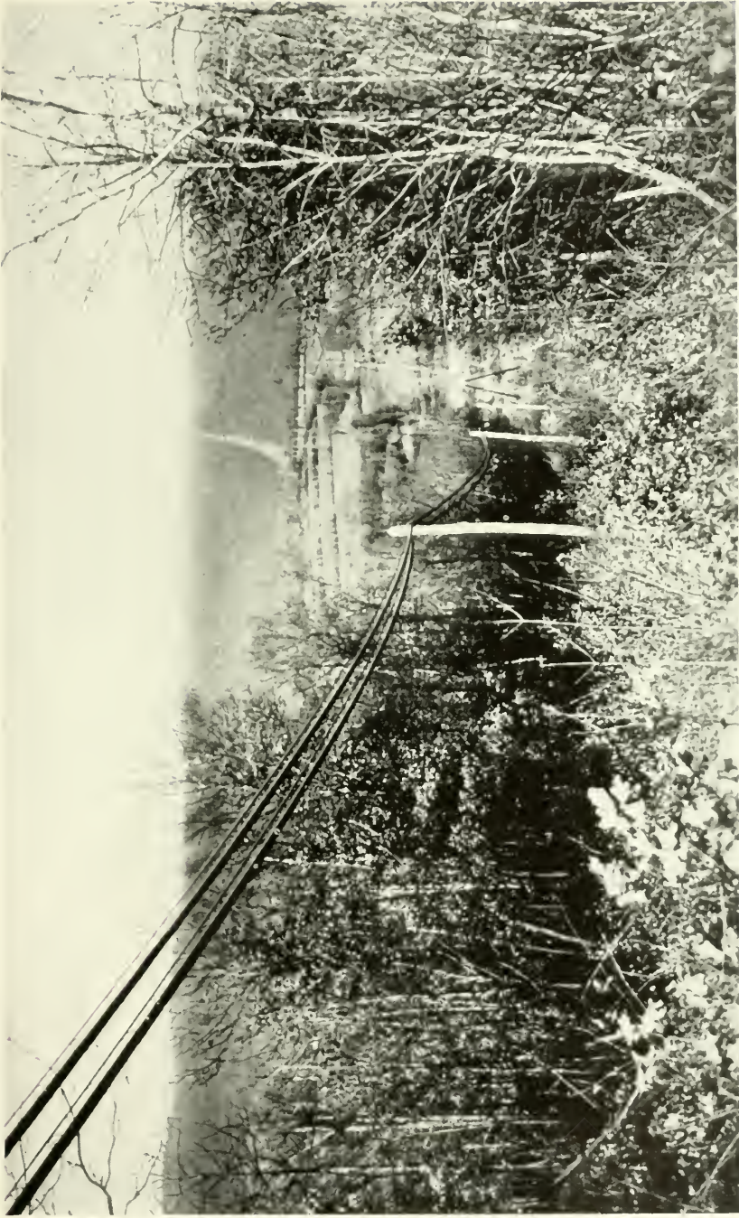
FIGURE 7. RADIO PROGRAMS GENERALLY TRAVEL THROUGH CABLE AS LONG AS THEY ARE EAST OF THE MISSISSIPPI RIVER. THESE "COVERED HIGHWAYS" AFFORD A HIGH DEGREE OF PROTECTION AGAINST WEATHER HAZARDS
