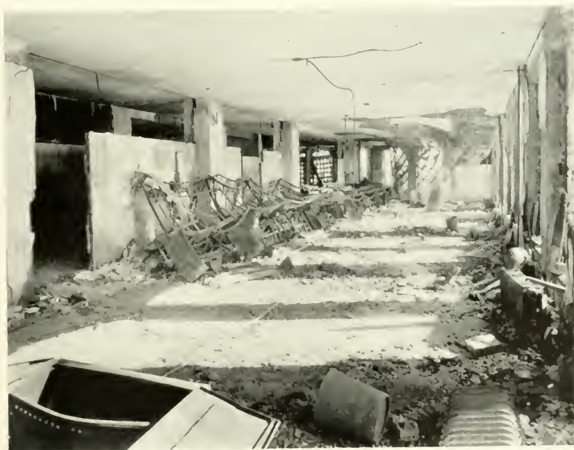
FIGURE 3. WHAT WAS LEFT OF THE LOCAL SWITCHBOARD IN ANDERSON ON THE MORNING OF JANUARY 29.
