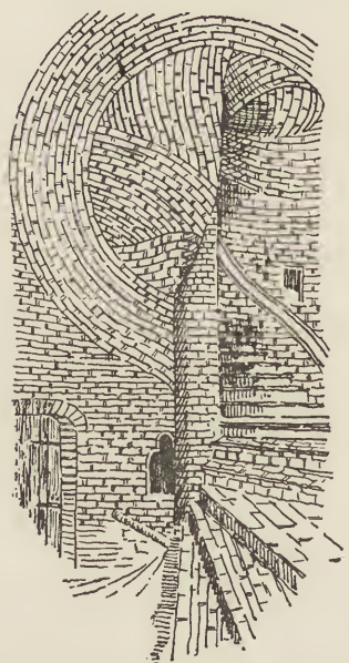
Staircase, House of Tristan the Hermit, Tours, France.
