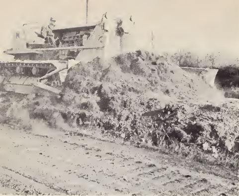
Municipal road-grading machinery in operation.
