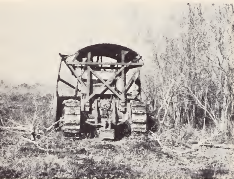
Clearing with modern equipment.
