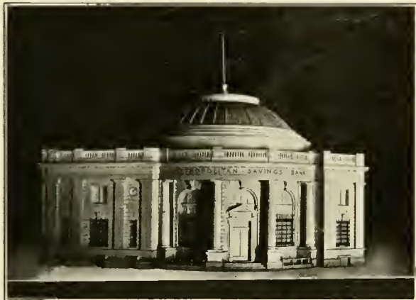
New Bank, in Course of Construction, S. W. Cor. Charles and Saratoga Sts.
