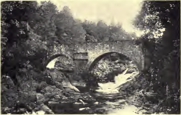
Bridge of Feugh
