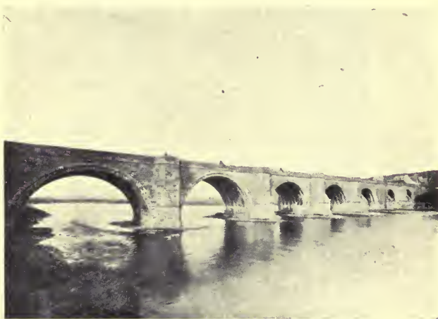
Old Bridge of Dee
