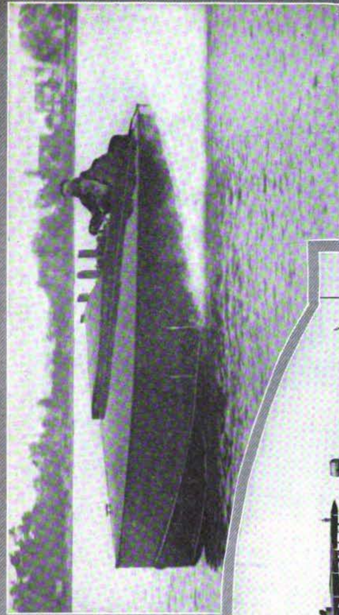
Tech, Jr., designed by Adolph Apel, for Coleman DuPont, which has already shown speeds of nearly 60 miles an hour. This boat will be a challenger for the Gold Cup, and is powered with an eight-cylinder 225 h.p. Sterling motor.
