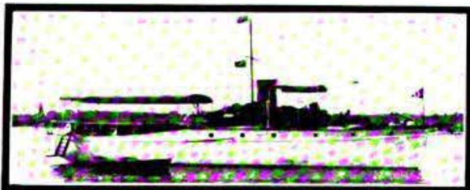
No. 1949.—Raised deck cruiser, 62 x 12.9; Sterling motor, heavy duty; deck controls.
