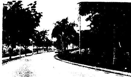
FIGURE 4. Airport Road is a bituminous surface, 4-lane divided highway (U/OU)
