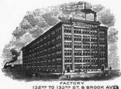
FACTORY 132 ND TO 133 RD ST. & BROOK AVE
